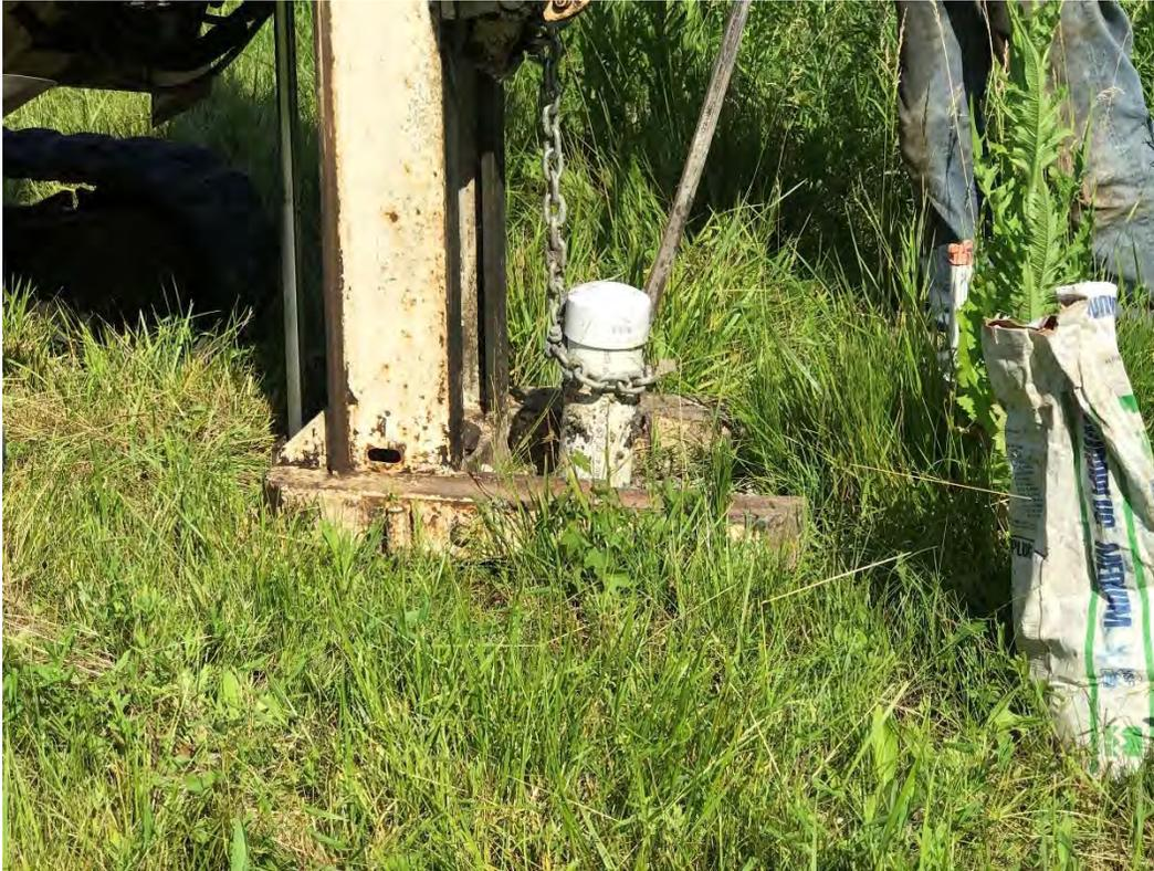
Next, the one-inch diameter PVC well screens and casings were removed from the ground with the assistance of the Geoprobe track rig (a chain was placed around the well and the hydraulic hammer from the track rig was used to pull the well out of the ground, see photo above). Tubing associated with the soil vapor probe was detached from the vapor probe and pulled from the ground.
