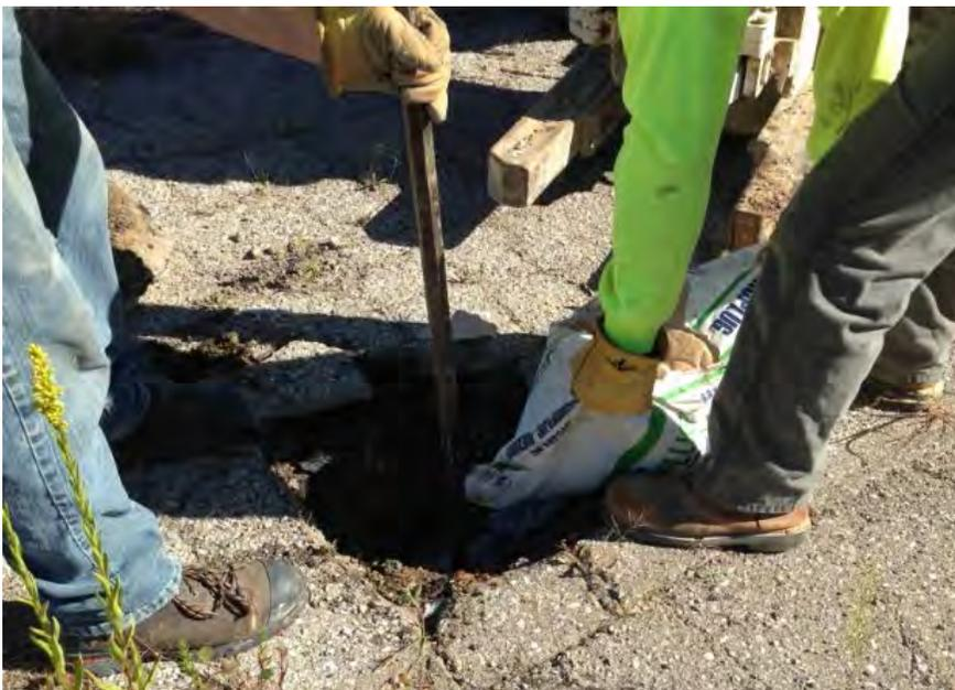
Finally, the surface at each location was restored to a similar condition. In the gravel covered areas, the final six inches were filled with gravel. In the asphalt area at OW-9, the final six inches were filled with concrete (see photo below).
