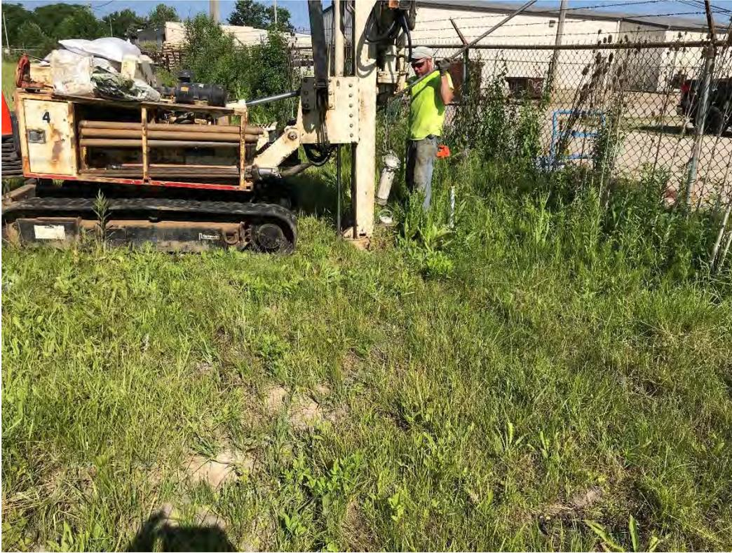
Then each borehole was sealed to the surface with bentonite chips and compacted with the breaking bar to prevent bridging.
