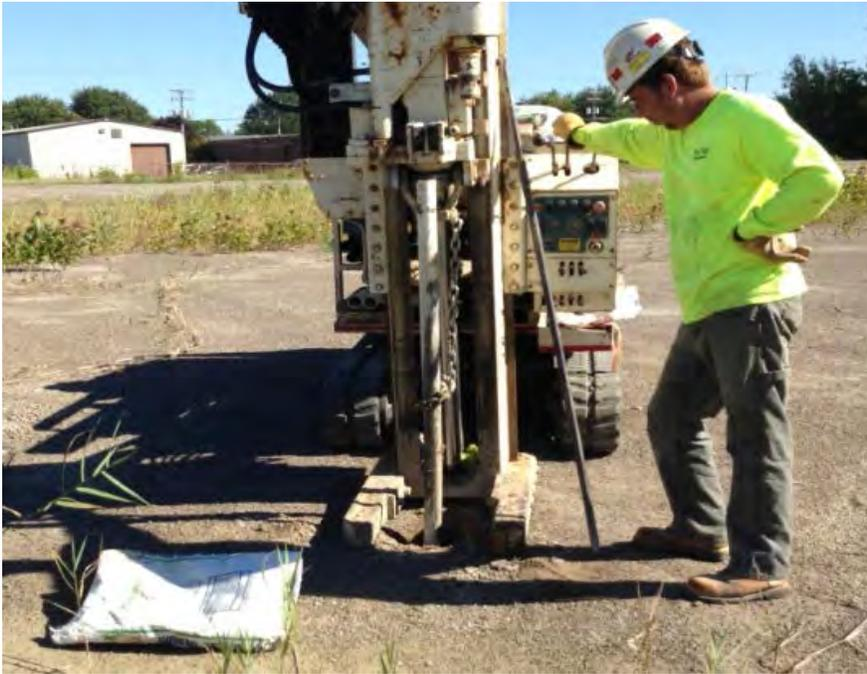
Then each bore hole was sealed to within six inches of the surface with bentonite chips and compacted with the breaking bar to prevent bridging (see photo below).
