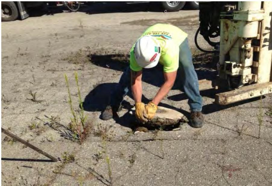
Next, the two-inch diameter PVC well screens and casings were removed from the ground with the assistance of the Geoprobe track rig (a chain was
