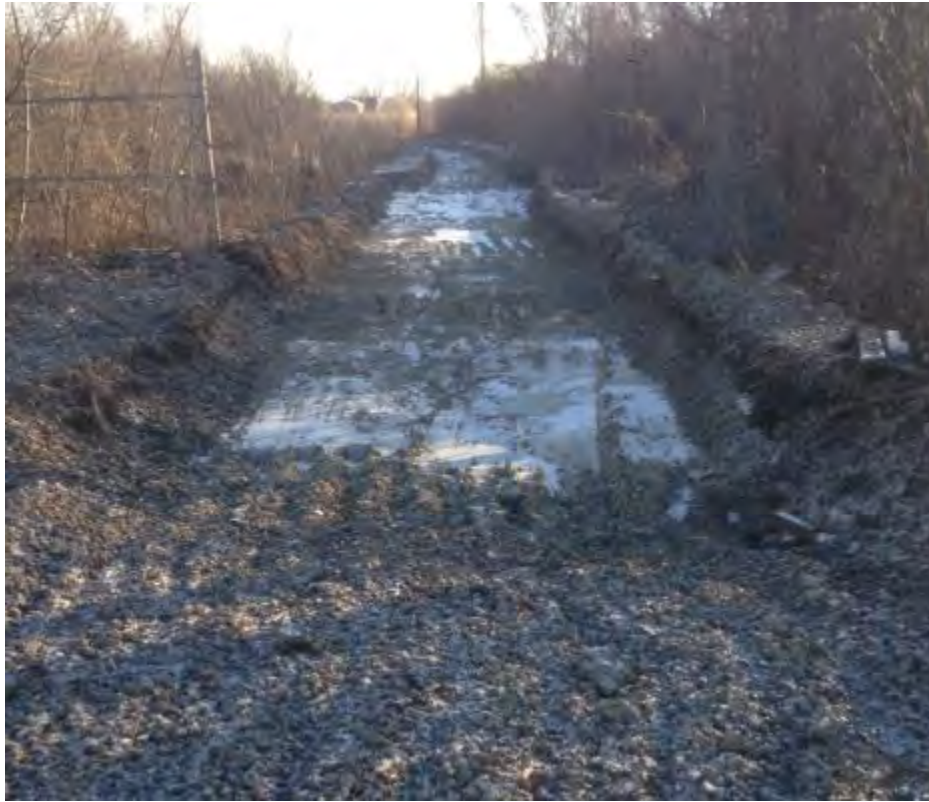
Photo 5 – View eastward along excavated rail spur on 5 January 2015 prior to restoration.
