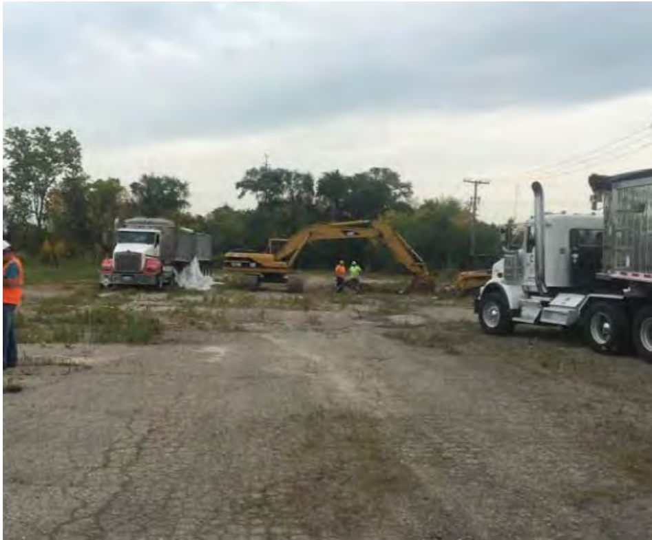
Photo 6 - View eastward towards ongoing Excavation #1B activities on 19 September 2017.
