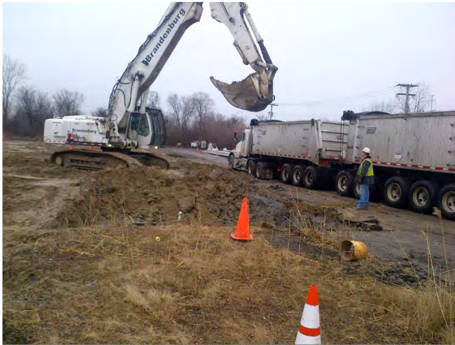
Photo 4 - Initiation of HWSB remedial excavation on 23 December 2014. View is eastward.
