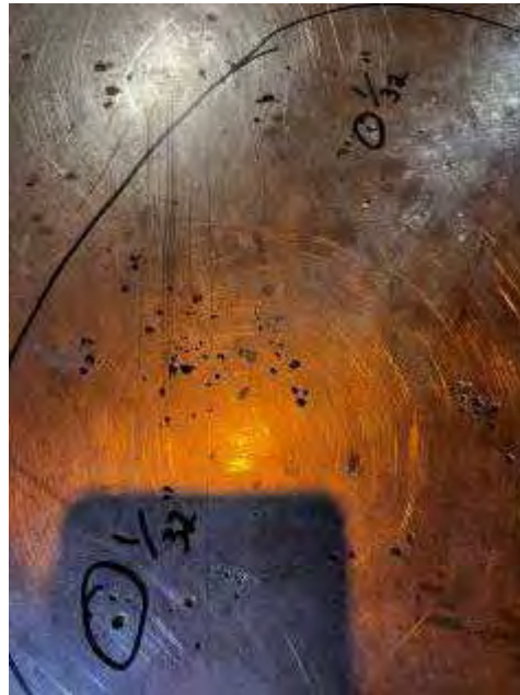
1/32" pitting on tank floor
