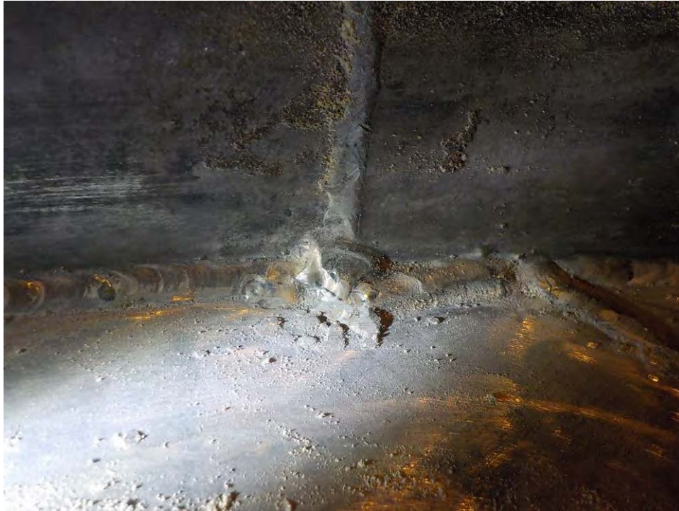
Example of the floor circumferential weld repairs with less than marginal weld quality and possible crevice corrosion
