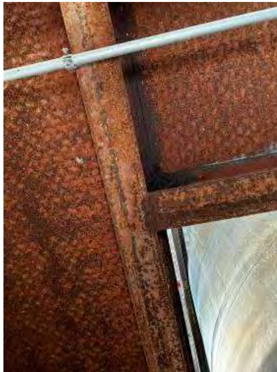
Catwalk I-beams displayed coating failures with active corrosion
