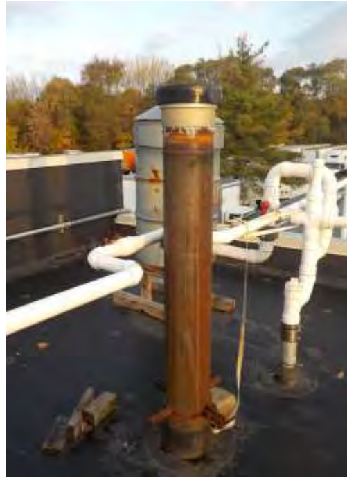
No protective coating observed on the external emergency vent piping
