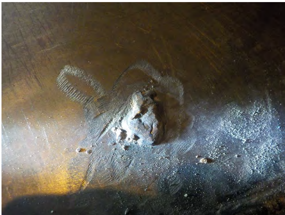
Example of puddle welding on the floor with possible crevice corrosion
