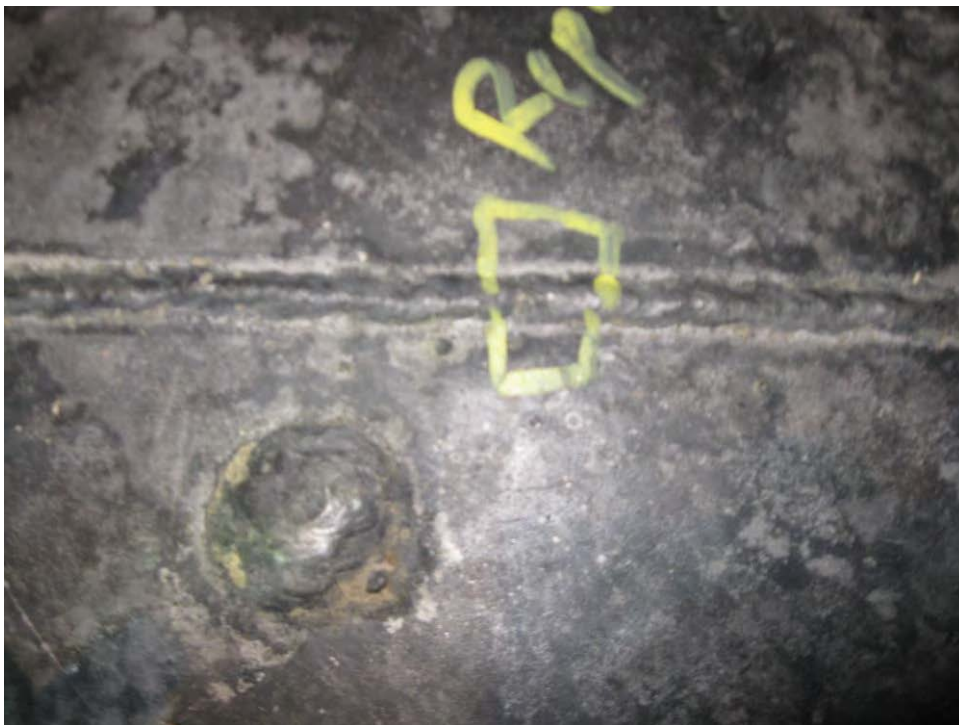
Pinhole noted on center seam weld
