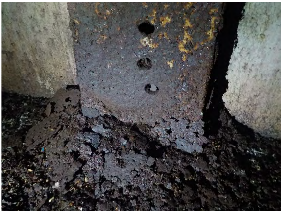
Corrosion from upper adjacent platform under containment
