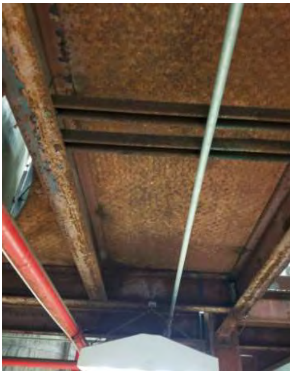
Catwalk supports with moderate corrosion
