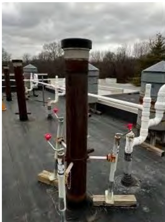
External emergency vent piping displayed no protective coating
