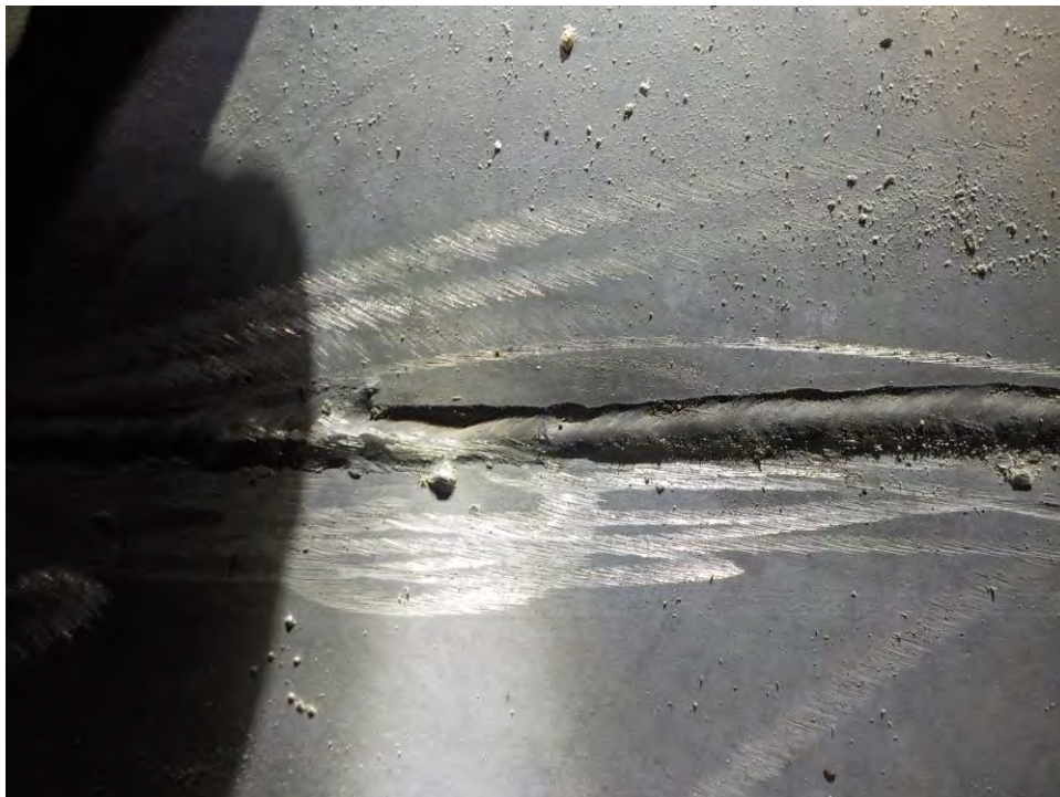
Floor seam weld with lack of filler metal and undercut
