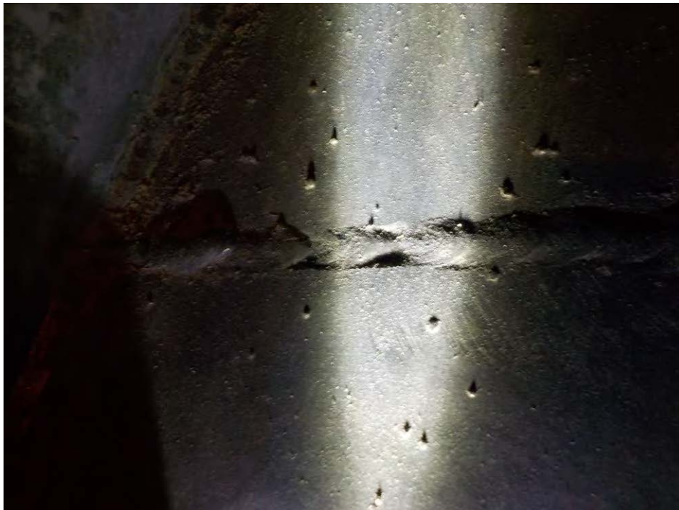
Floor seam weld with lack of filler metal and weld spatter
