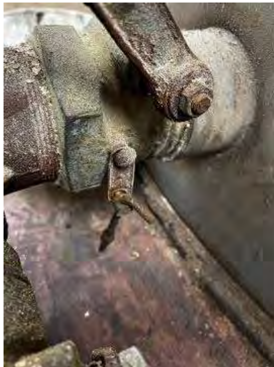
Mechanical damage noted on the fire valve fusible link
