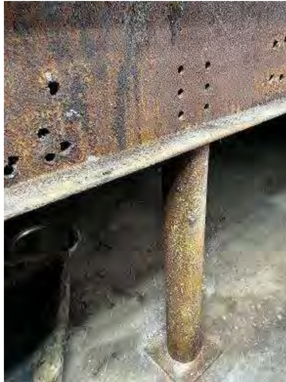
South floor supports displayed coating failures with active corrosion
