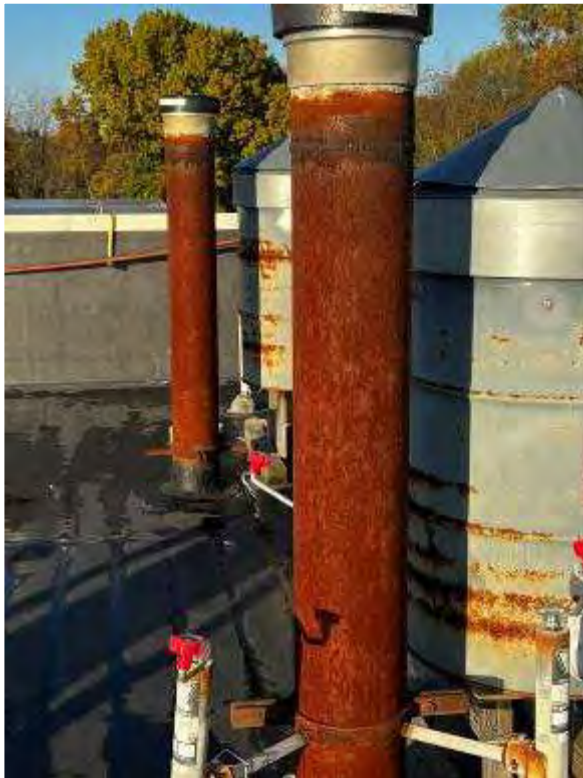
E-Vent piping displayed no protective coatings
