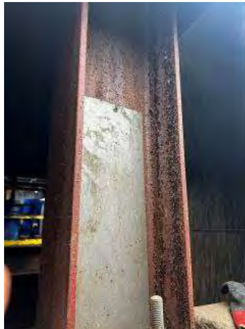
Coating failure observed on the I-beam supports with active corrosion
