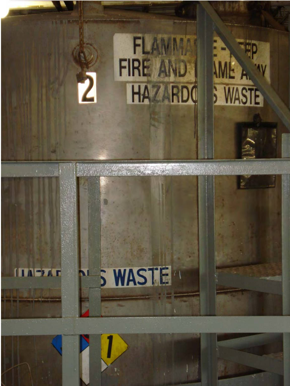
NFPA Markings on Tank #2
