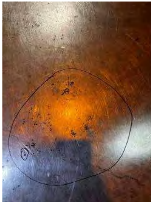
1/32" pitting on tank floor
