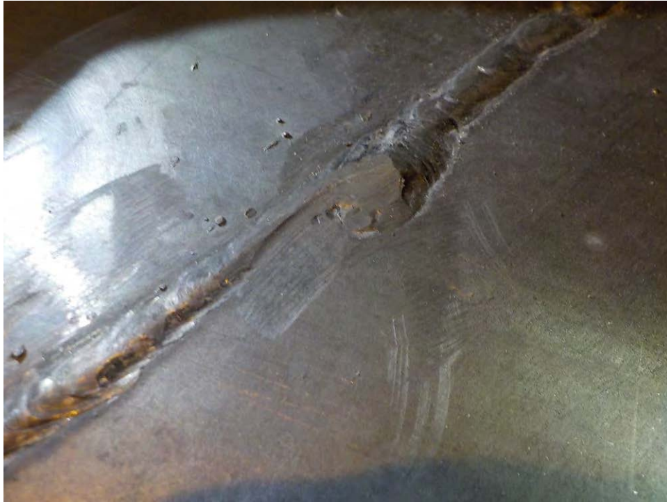
Floor seam weld repair with lack of fill and possible crevice corrosion
