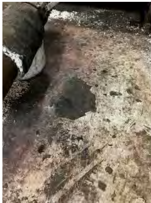
Containment floor displayed coating failures
