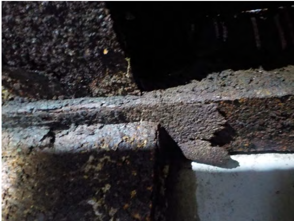
Significant corrosion under support structure located under containment
