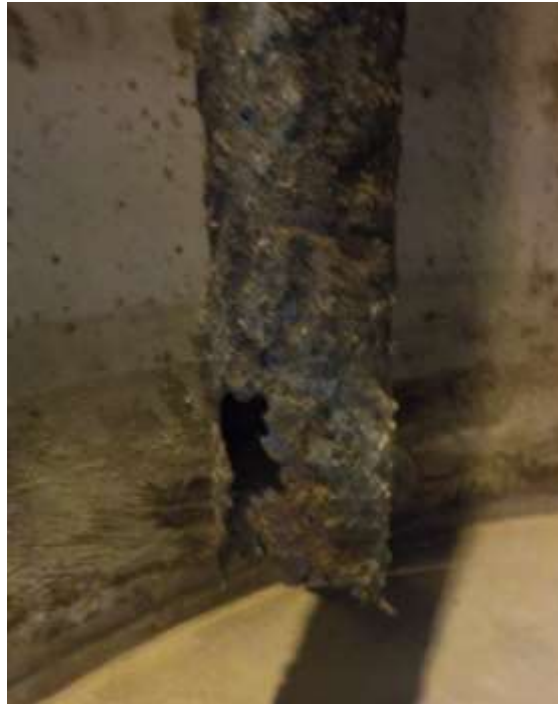
Inlet piping is severely corroded
