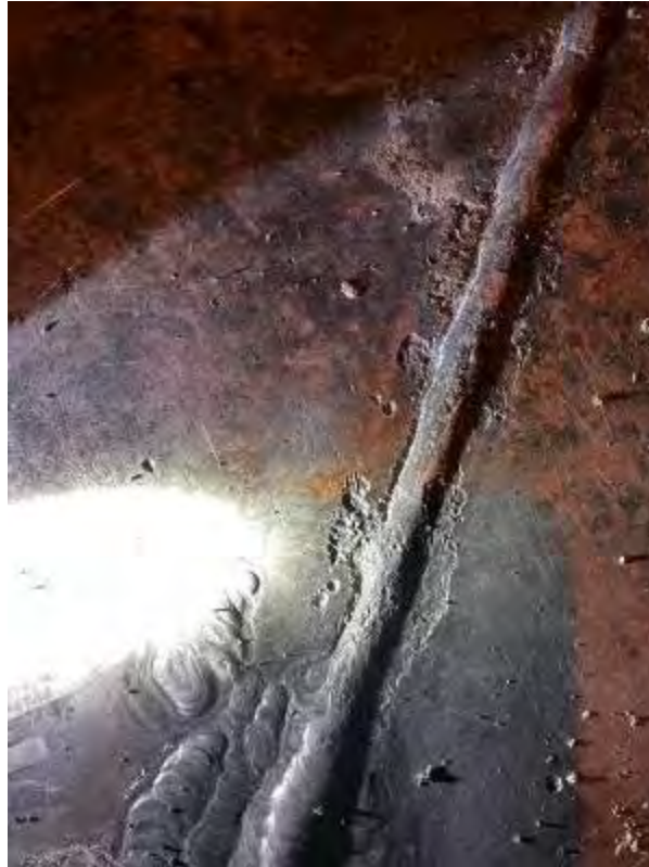
Example of uniform 1/16" pitting noted on the floor
