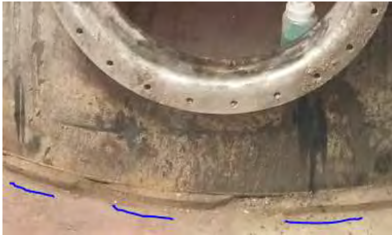
Wood planks beneath Tank
