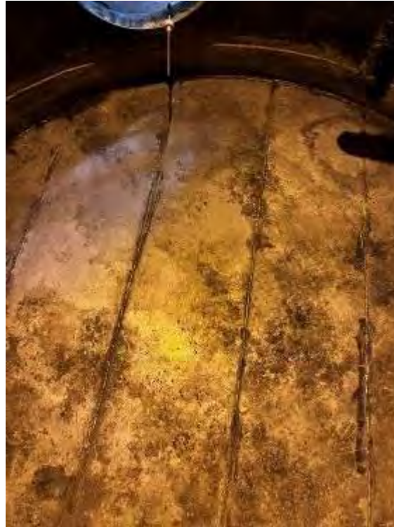
General picture of tank floor
