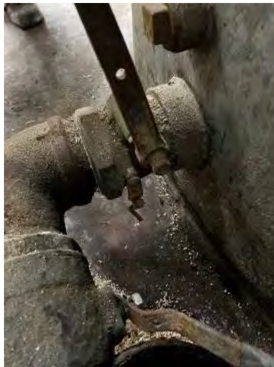
Fire valve was disconnected at time of inspection
