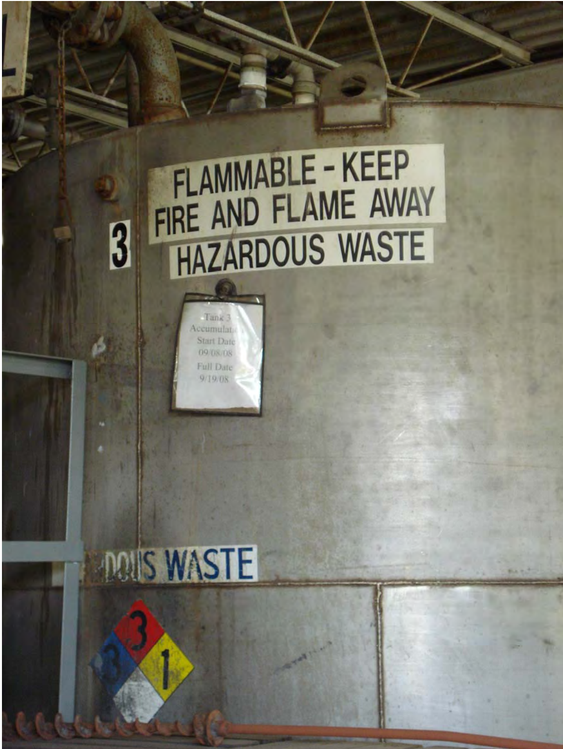
NFPA Markings on Tank #3
