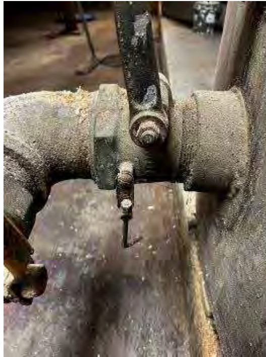
Fire valve at nozzle N-1 was disconnected at time of inspection
