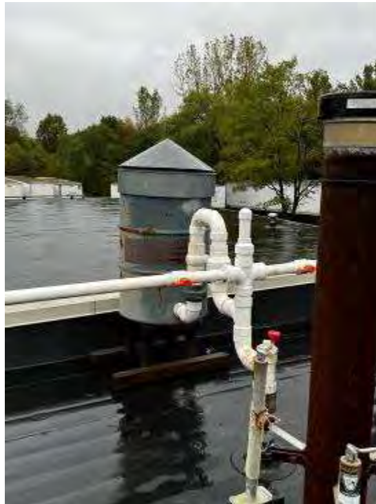
Sample port in conjunction with normal venting without 2 hour fire rating material
