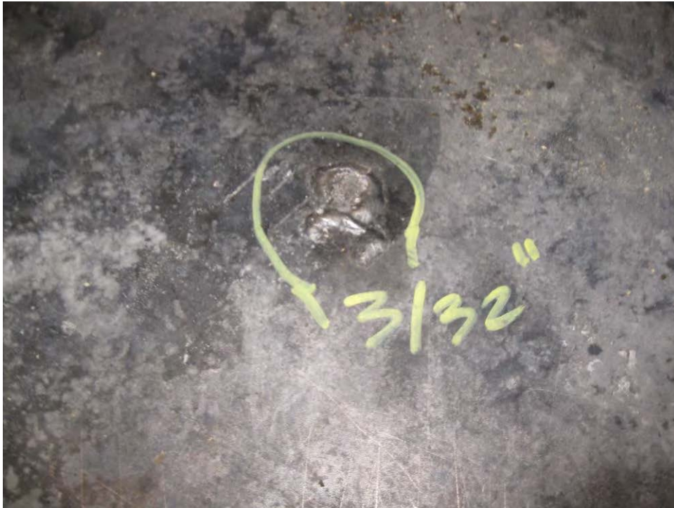
Previous weld repair has deteriorated causing a 3/32" pit
