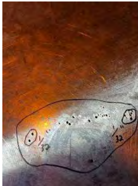
1/32" pitting on tank floor
