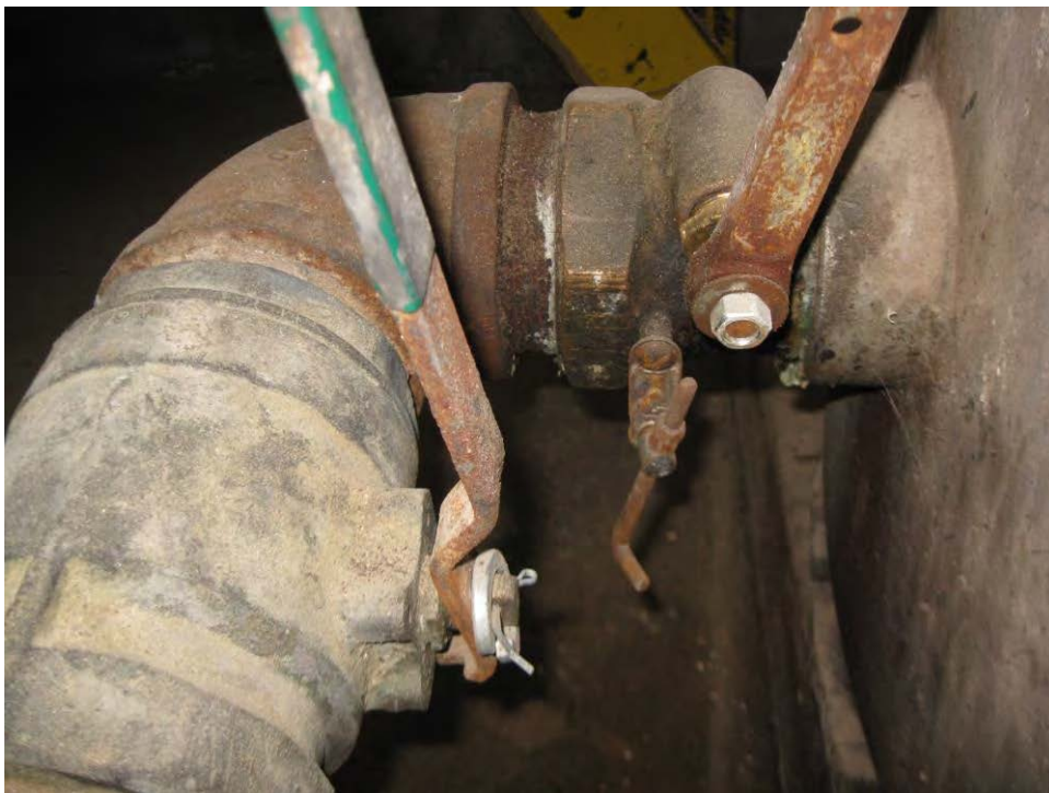
Fusible fire valve was disconnected at time of inspection
