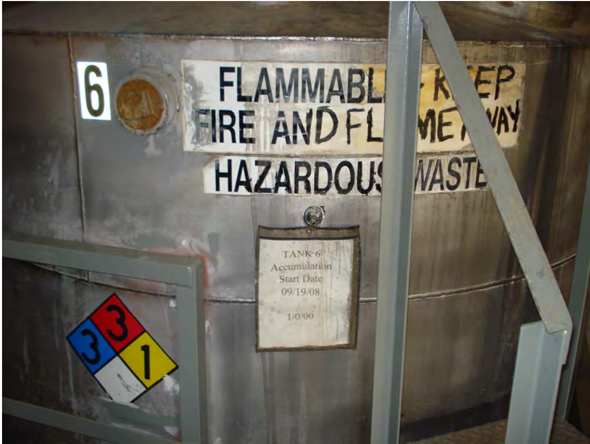
NFPA Markings on Tank #6
