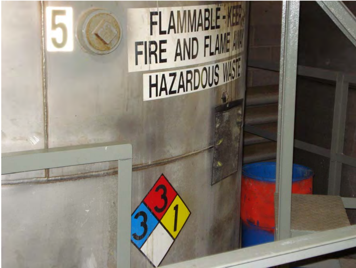
NFPA Markings on Tank #5
