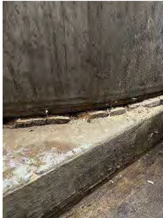
Tank is elevated on no-fire rated material
