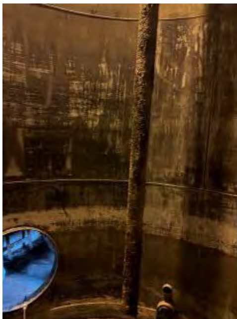
Dip tube inside of tank is badly corroded with through wall holes
