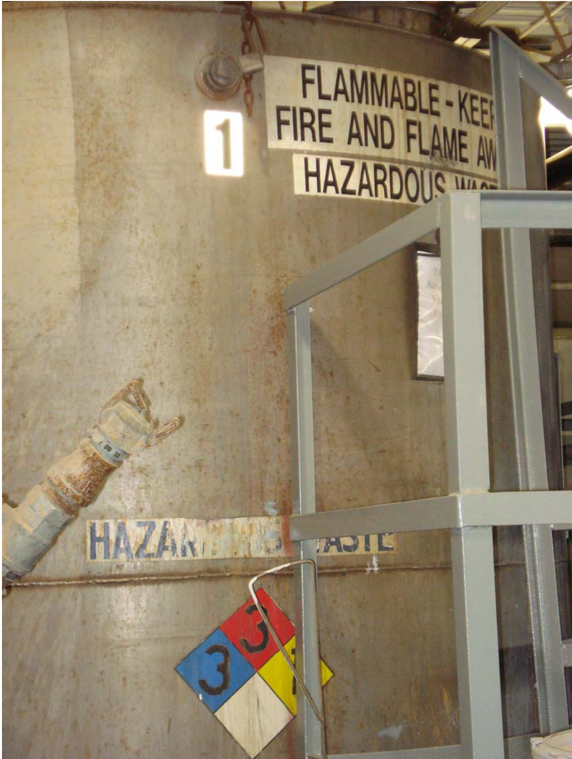
NFPA Markings on Tank #1
