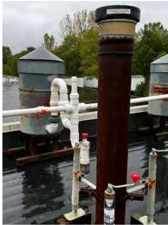
Coating failures observed on external emergency vent piping
