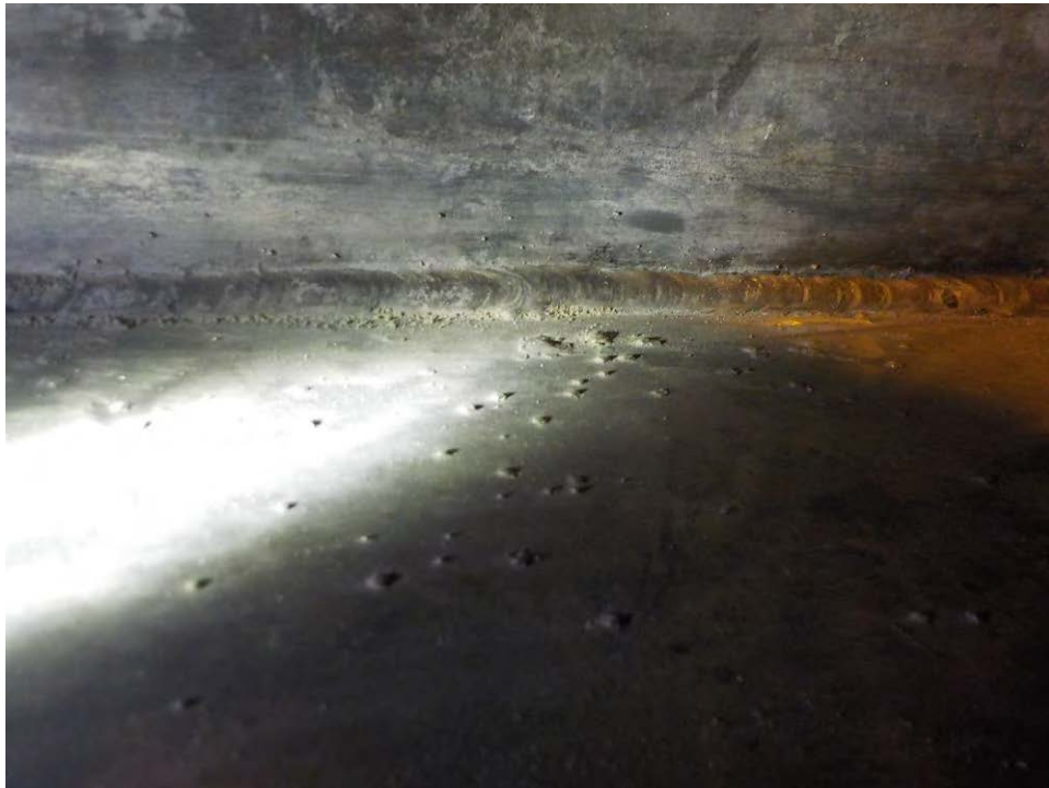
Weld spatter observed in the floor
