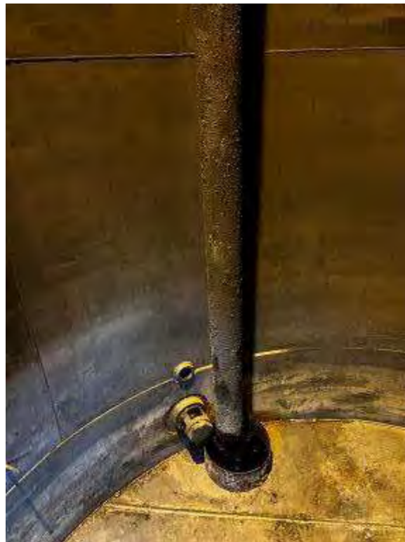
Internal dip tube
