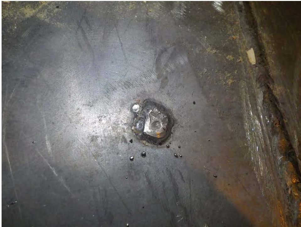
Example of puddle welding performed on the floor with weld spatter and possible crevice corrosion
