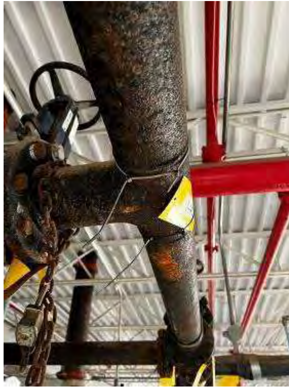
Coating failures with active corrosion noted on associated feed piping
