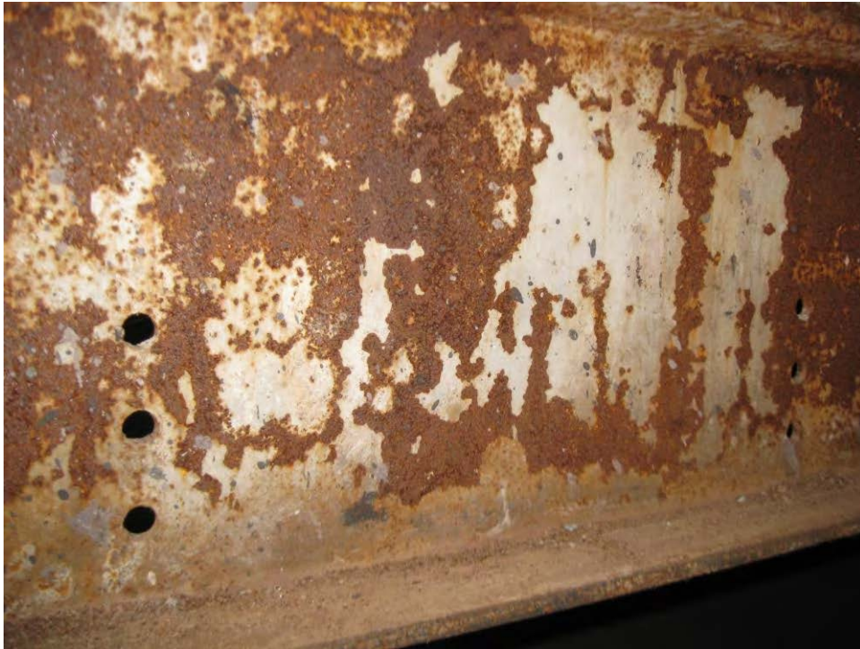
I-beam supports for platform displayed coating failures with active corrosion
