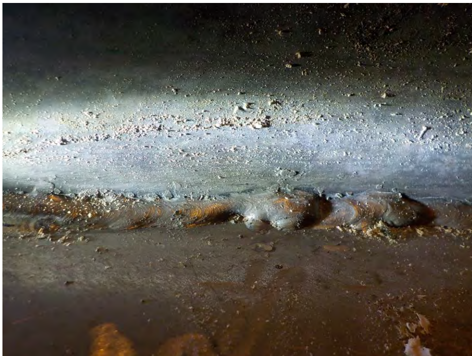
Example of floor to reinforcement band fillet weld with poor weld quality
