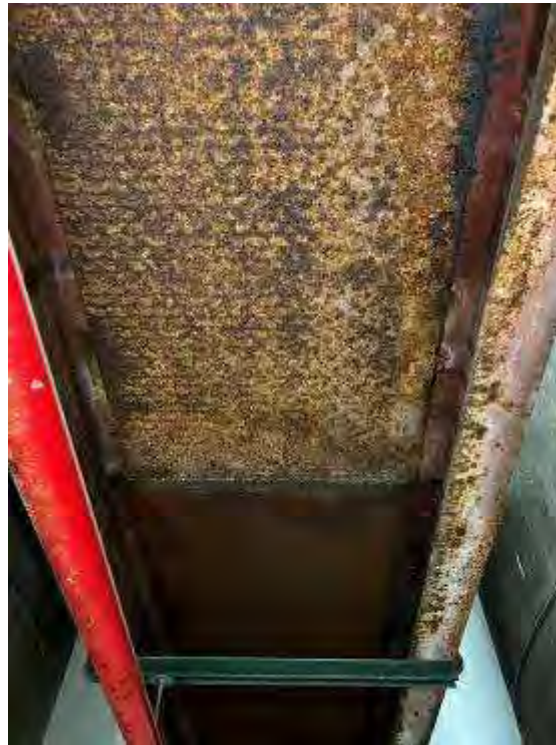
Coating failures with active corrosion noted on the platform supports and diamond plating
