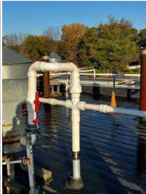
PVC Piping being utilized instead of two hour fire rated material
