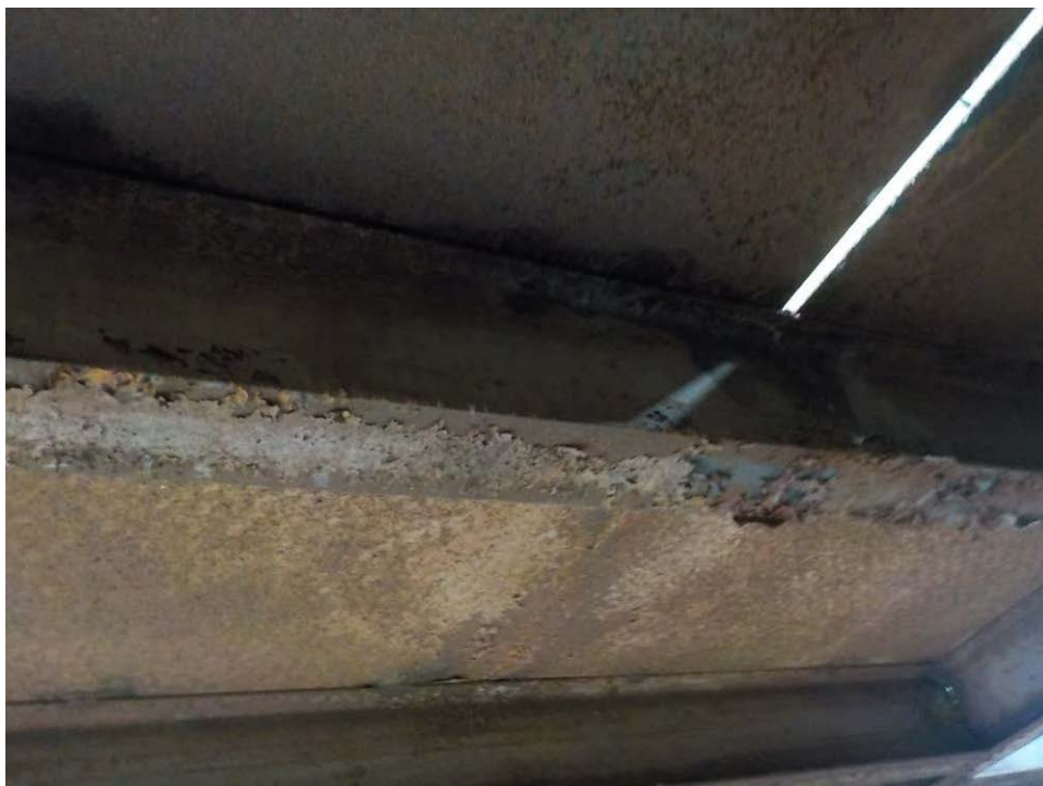
Surface corrosion observed on supports and underneath catwalk
