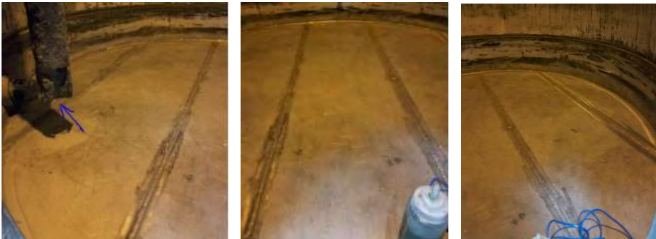
New Tank Floor with perimeter ring Note corroded inlet piping (Left Photo)
