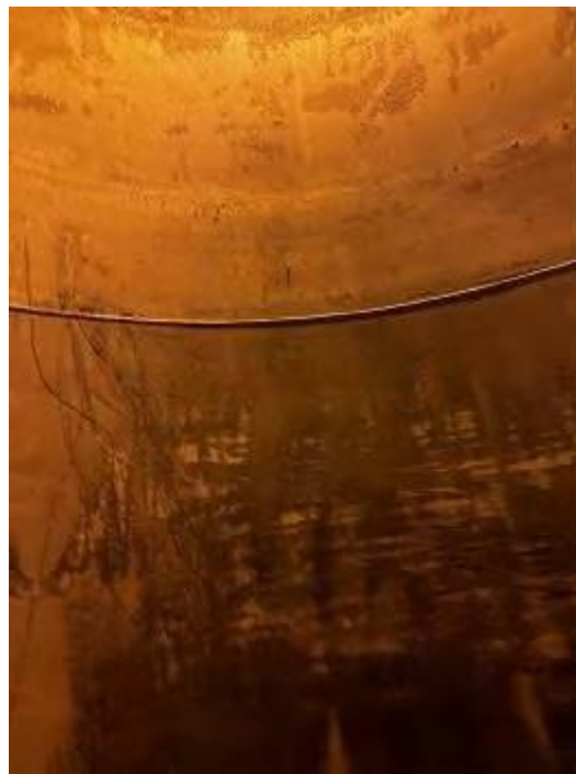
General picture of tank shell
