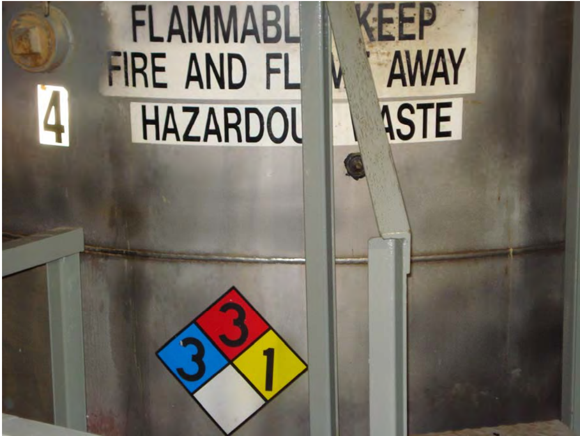
NFPA Markings on Tank #4
