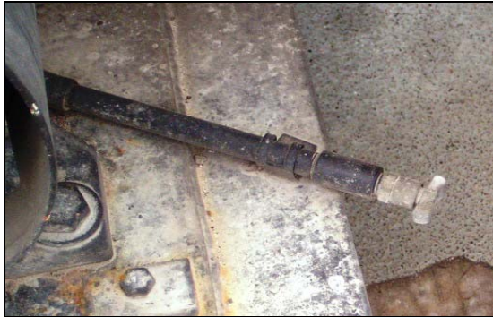
Picture 10 – Drain valve on vac pump
