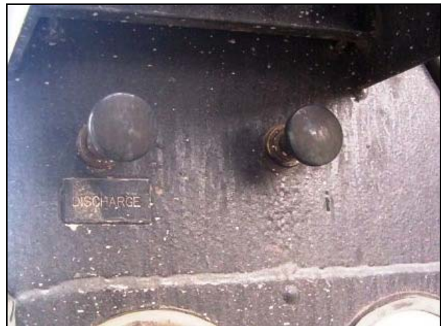
Picture 4 – Air operated valves
