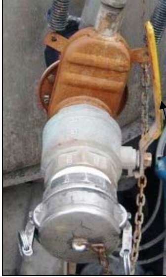
Picture 9 – Inlet brass secondary valve
