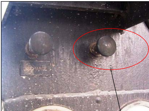
Picture 2 – Intake switch
