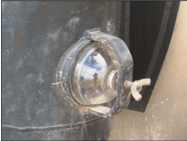
Picture 1 – Sight glass on trap tank
