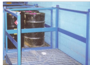
Example of using racks to protect drums from physical damage from
