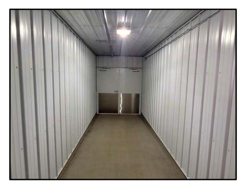
View of Recessed Floors for Secondary Containment in Connecting Corridors
