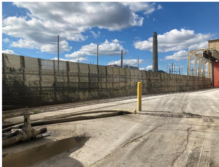
Figure 24. Splashguard on Northwest Boundary of Site
