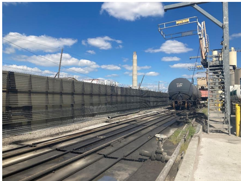
Figure 23. Splashguard on Southwest Boundary of Site
