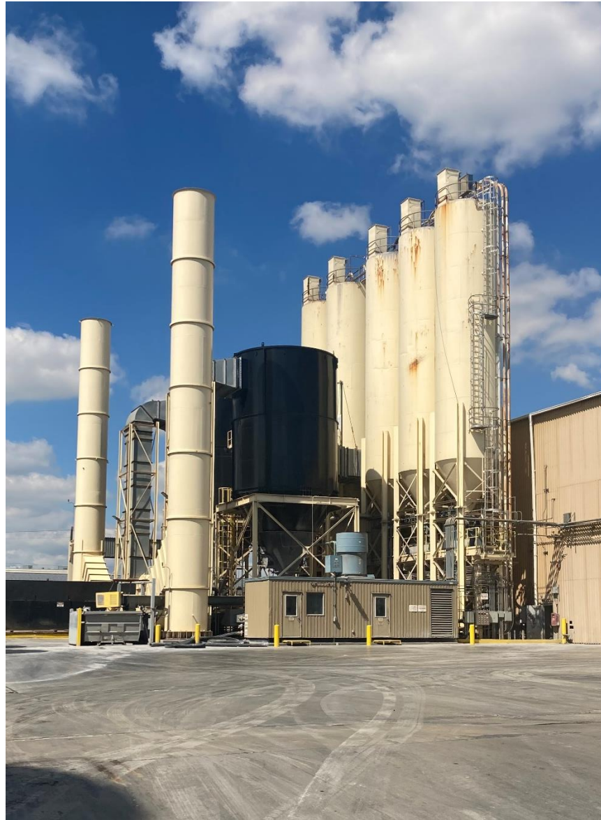
Figure 25. S-1, S-2, S-3, S-4, H-1 and Chem Fix Air Pollution Control System
