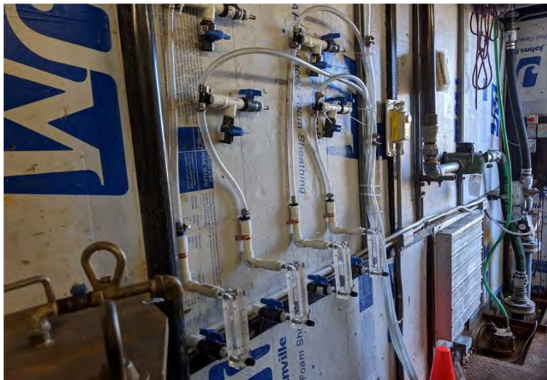
Photo 4: Influent manifold including flow meters and sampling ports
