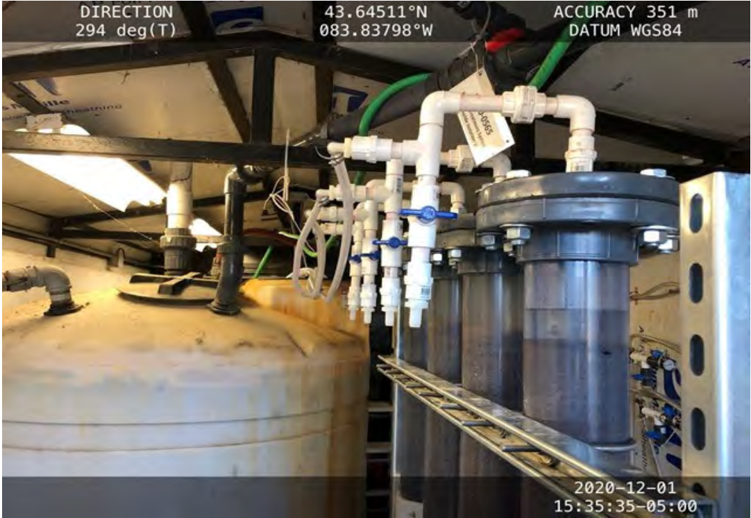
Photo 6: Effluent manifold and sample ports
