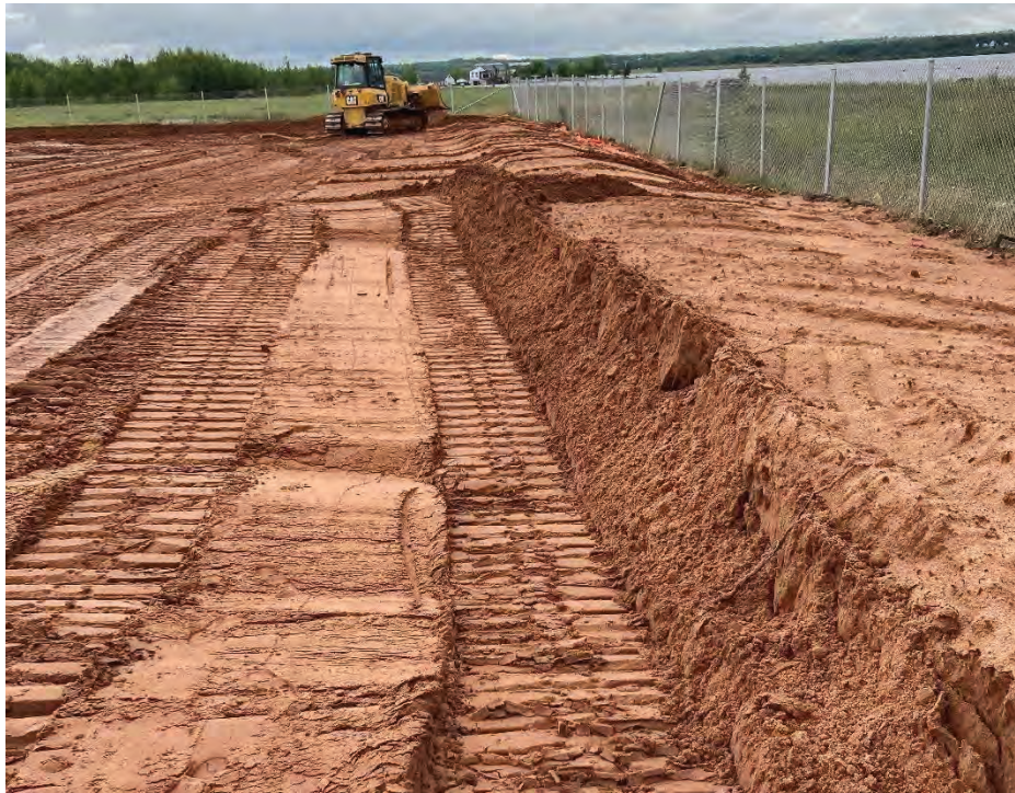
Forming the perimeter berm in the subgrade (facing north-northeast) 2020
