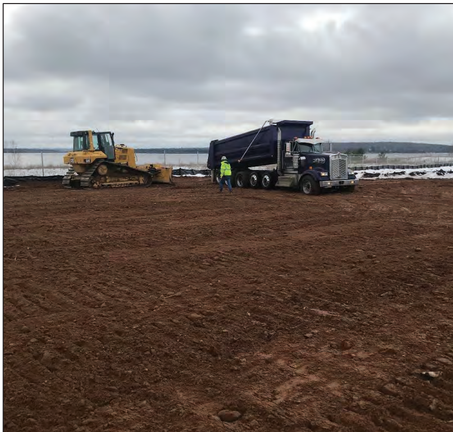
Load of sand delivered and placed in former WP-48 excavation (facing South) 2019
