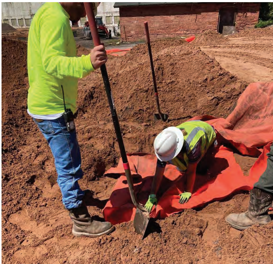
Repairing bulldozer tear in the demarcation fabric (facing northwest) 2020
