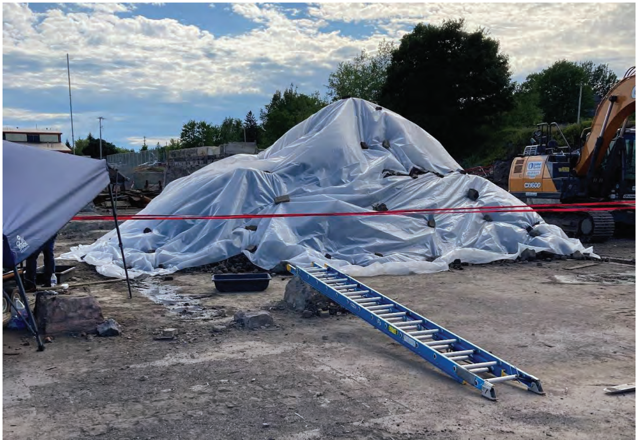
Stack Debris area material stockpiled, treated, sampled and covered awaiting disposal (facing west) 2020
