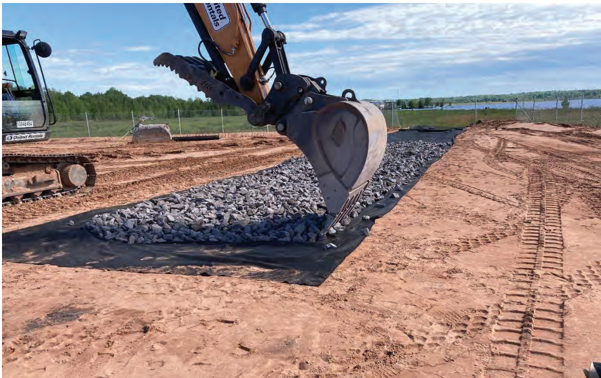
Constructing a swale in the eastern corner of the Site (facing east) 2020
