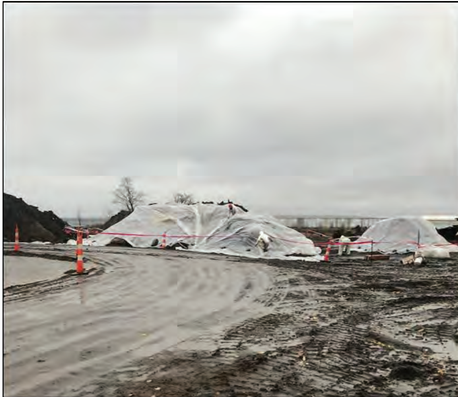
Covered non-hazardous with asbestos soil staging/load out area (facing Southeast) 2019
