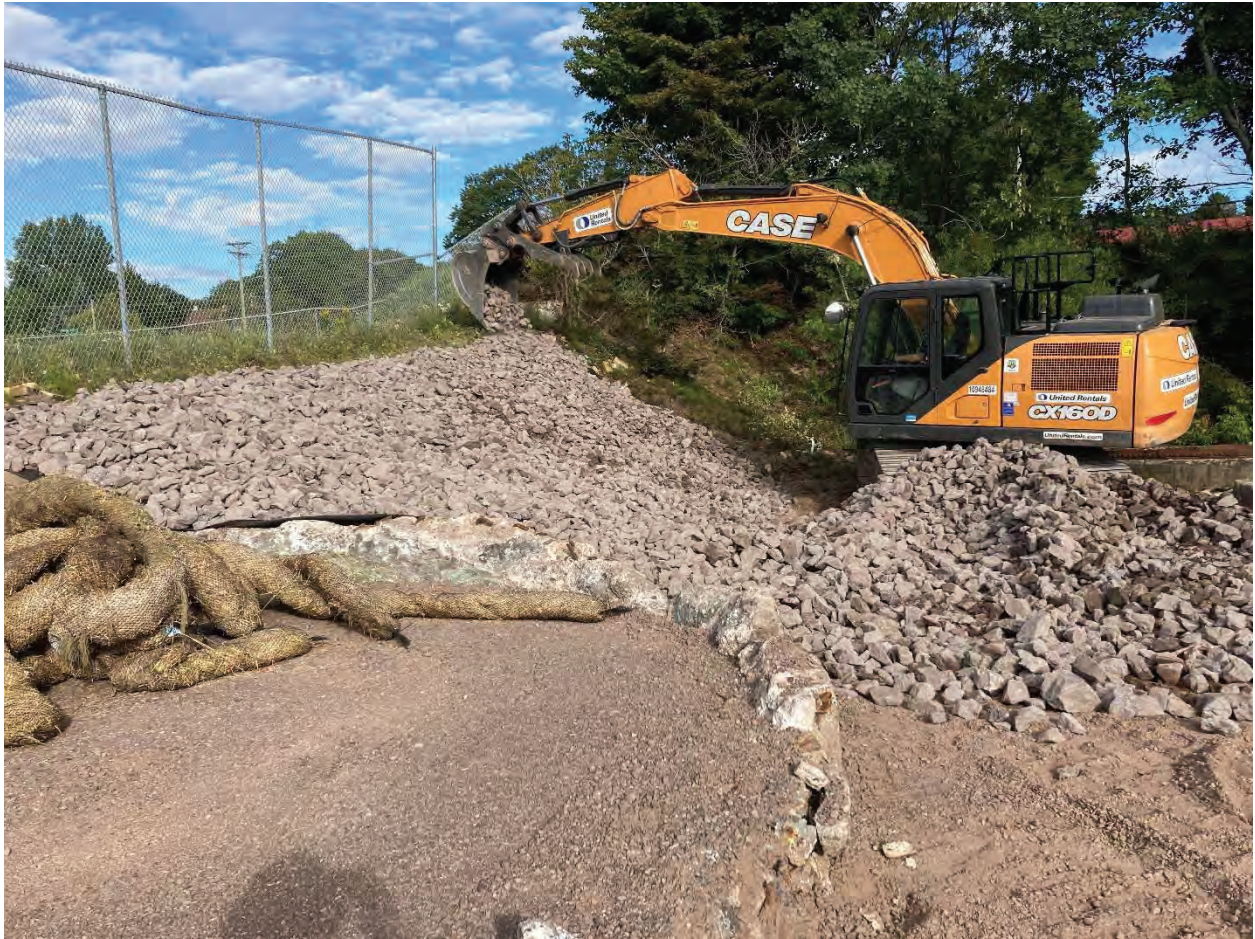
Placing riprap over geotextile fabric on the slope at the southwest corner of the Stack Debris area (facing west) 2020
