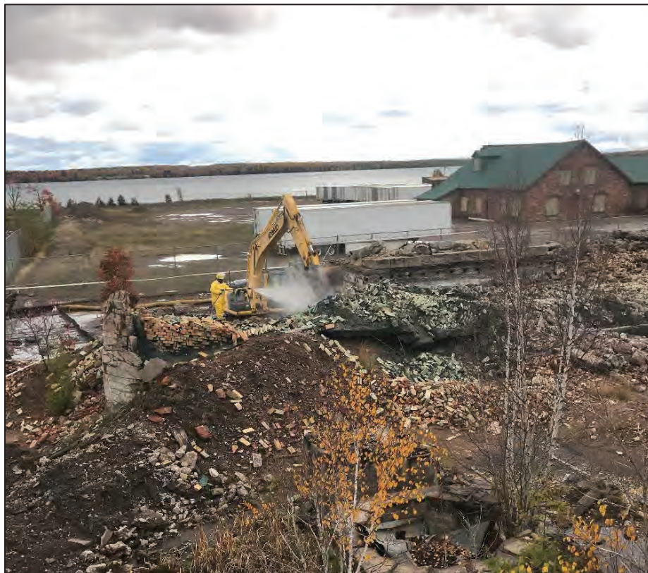
Dust suppression in the Stack Debris area (facing south) 2019
