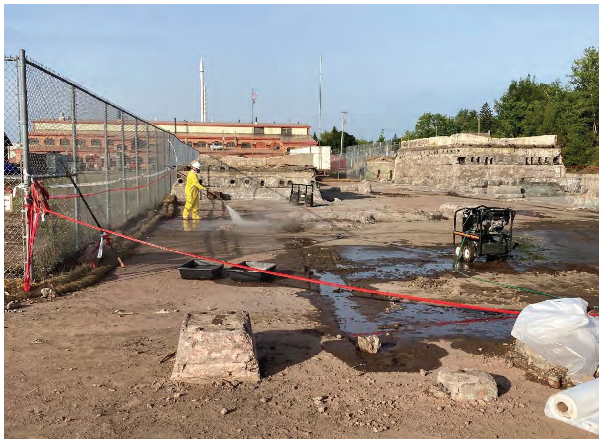
Washing Stack Debris Area where non-hazardous material with asbestos and EnviroBlend® was staged (facing southwest) 2020
