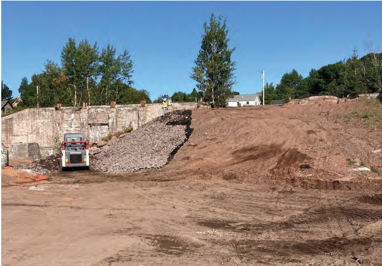
Placing riprap over geotextile fabric on the slope greater than 3 to 1 on the consolidation pile (facing west) 2020
