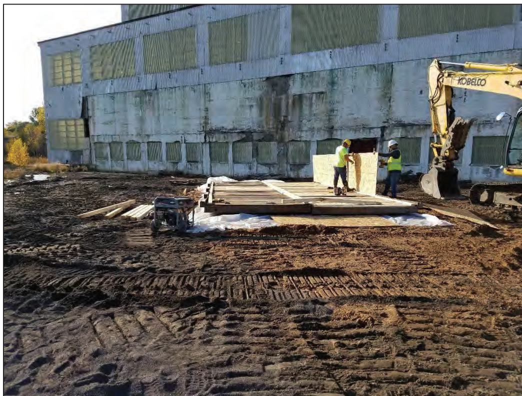
Decontamination pad construction (facing West) 2019
