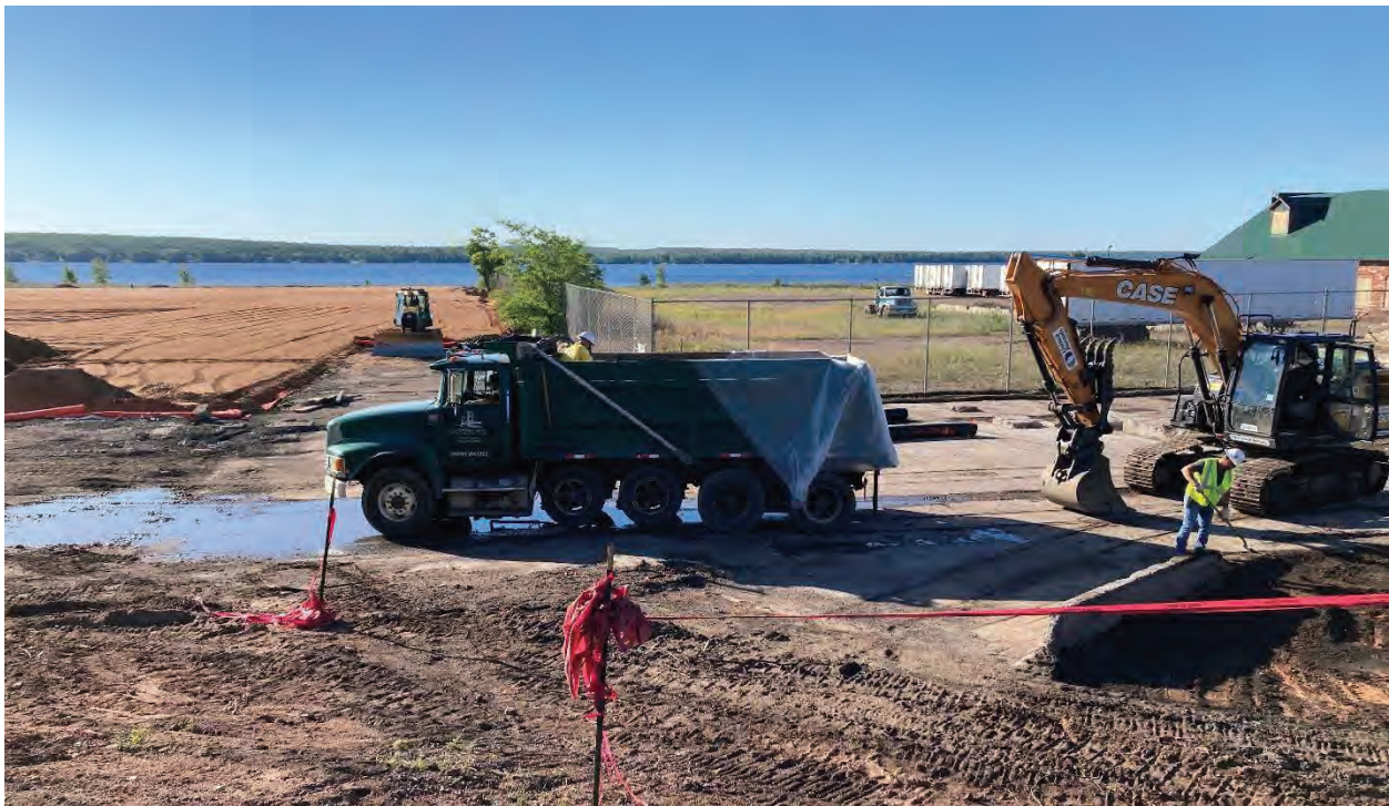
Final load of non-hazardous material with asbestos and EnviroBlend being sealed prior to leaving the Site (facing southeast) 2020
