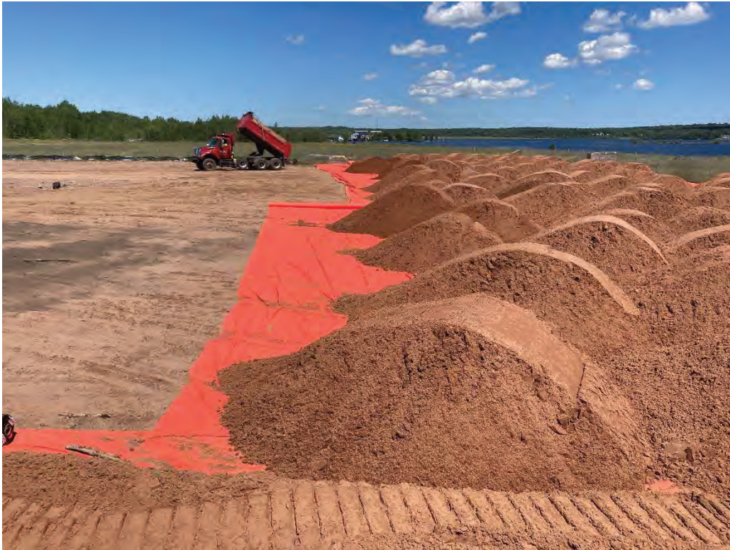
Importing sand as general fill over the demarcation fabric (facing northeast) 2020
