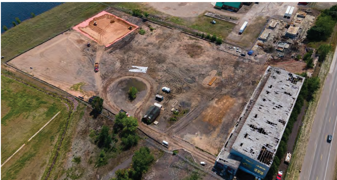
Aerial of site (facing south) as the demarcation fabric roll out and sand cover begins
