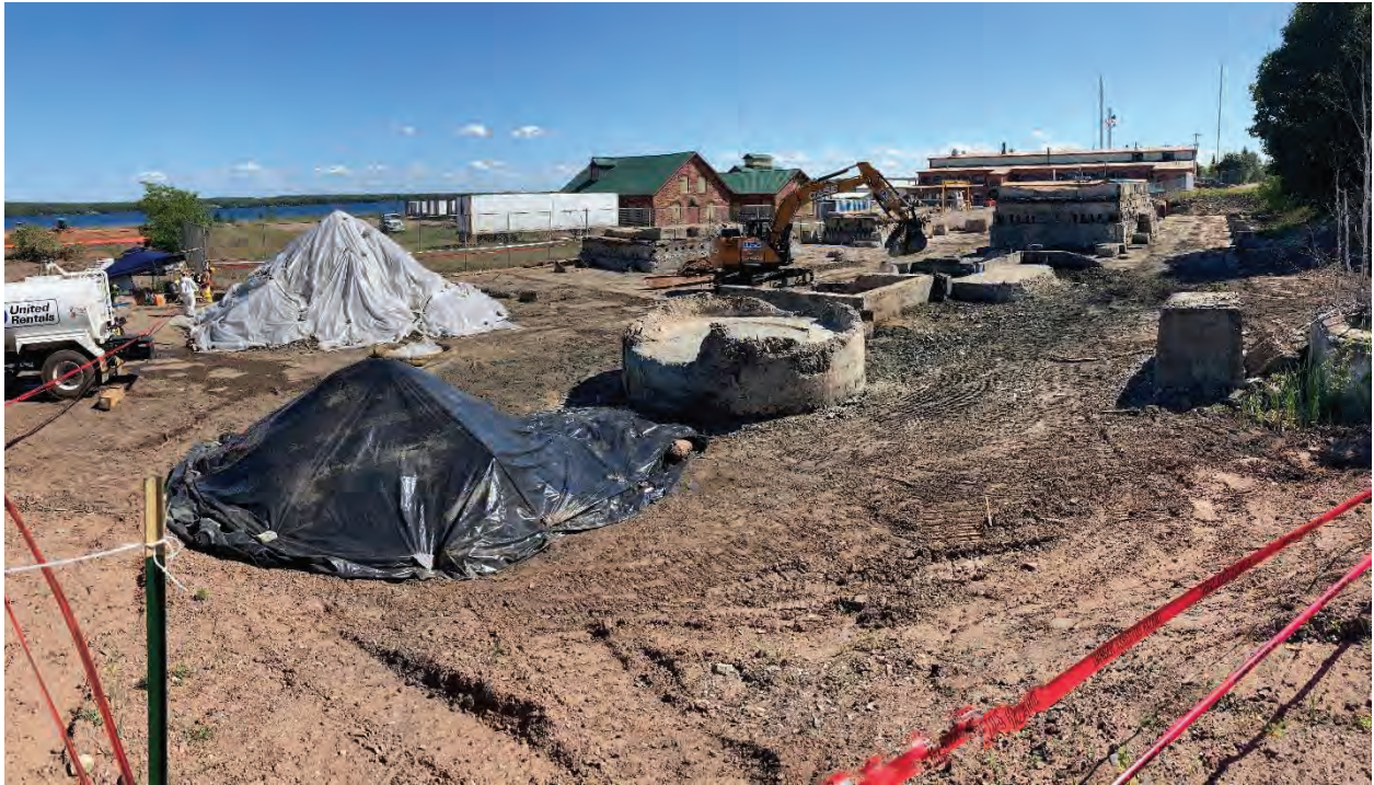
Hazardous Material from the stack bases has been stockpiled and covered awaiting disposal (facing south) 2020
