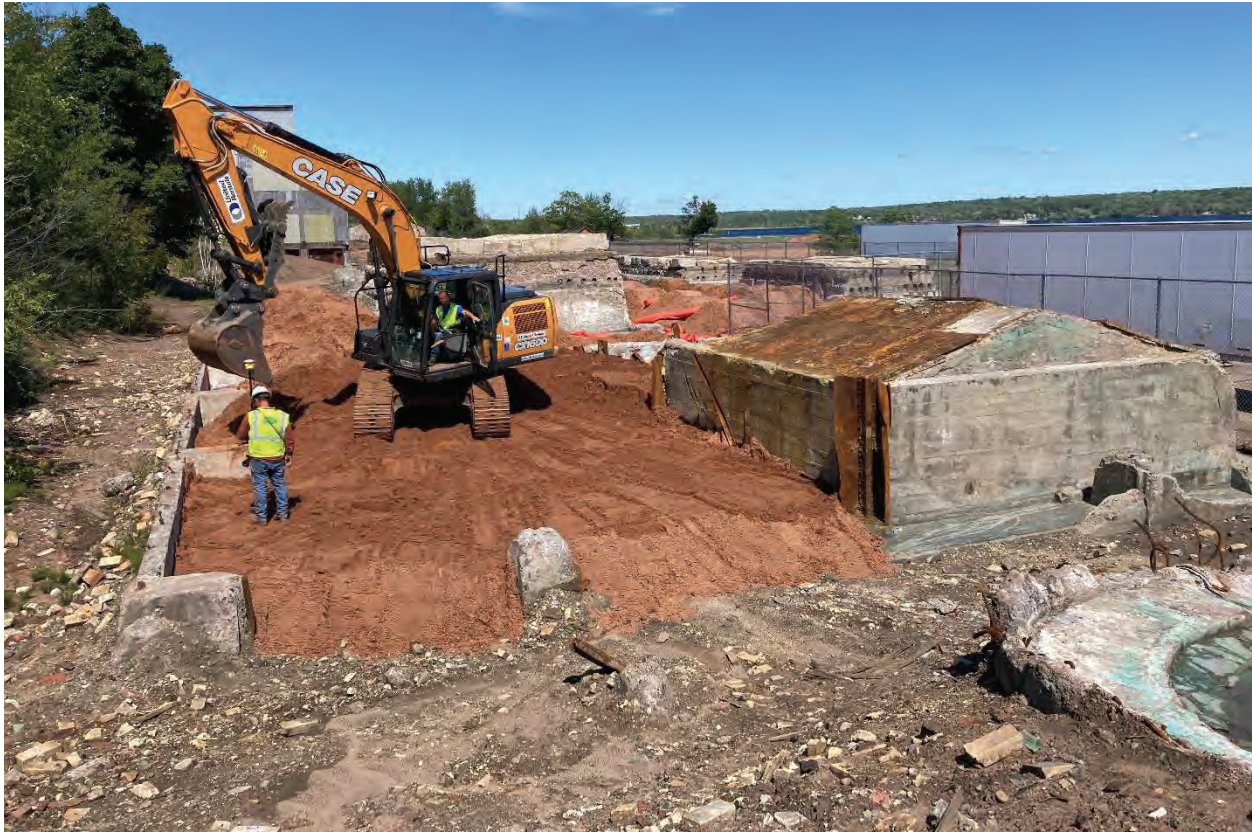
Place sand over demarcation fabric in the Stack Debris area (facing northeast) 2020
