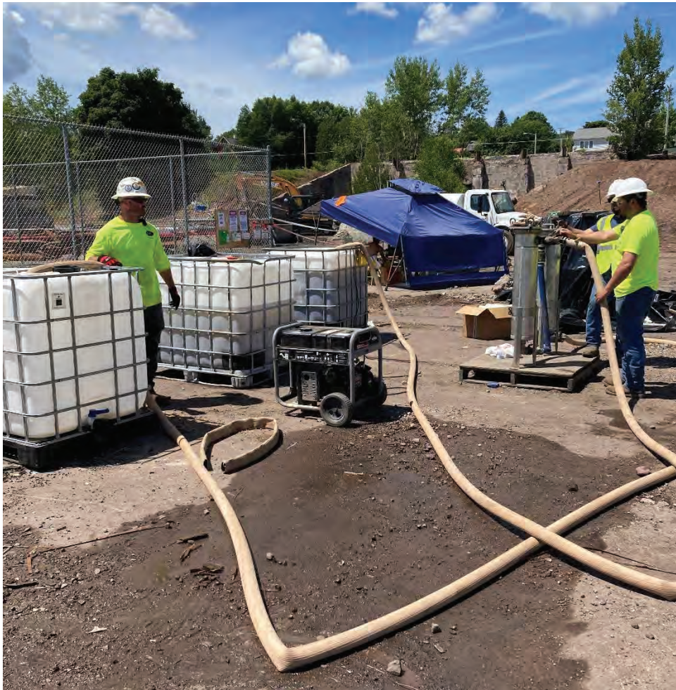
Filtering collected decontamination water (facing west) 2020
