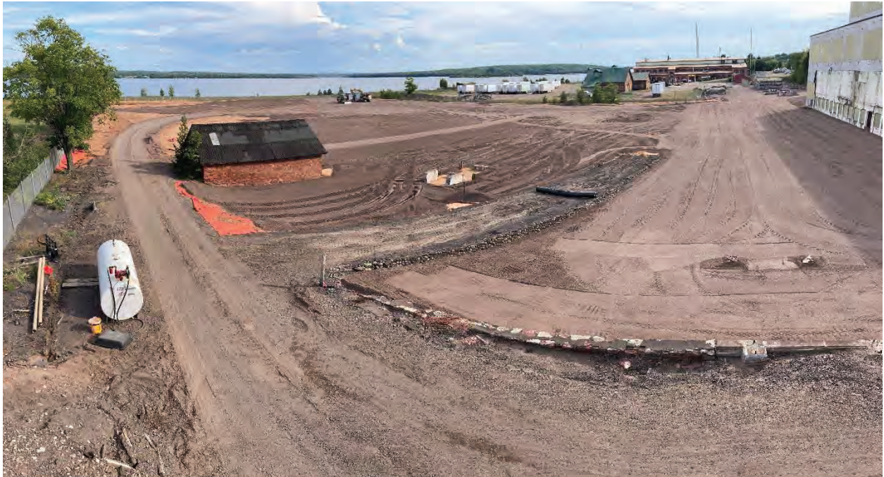
Sand placed and much of the 22A placed on the Site (panorama facing southeast to south) 2020
