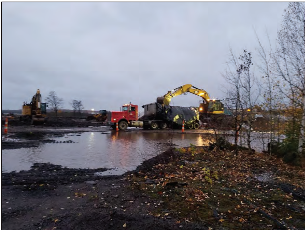
Lined truck being loaded with non-hazardous with asbestos material to be hauled to the landfill (facing South) 2019
