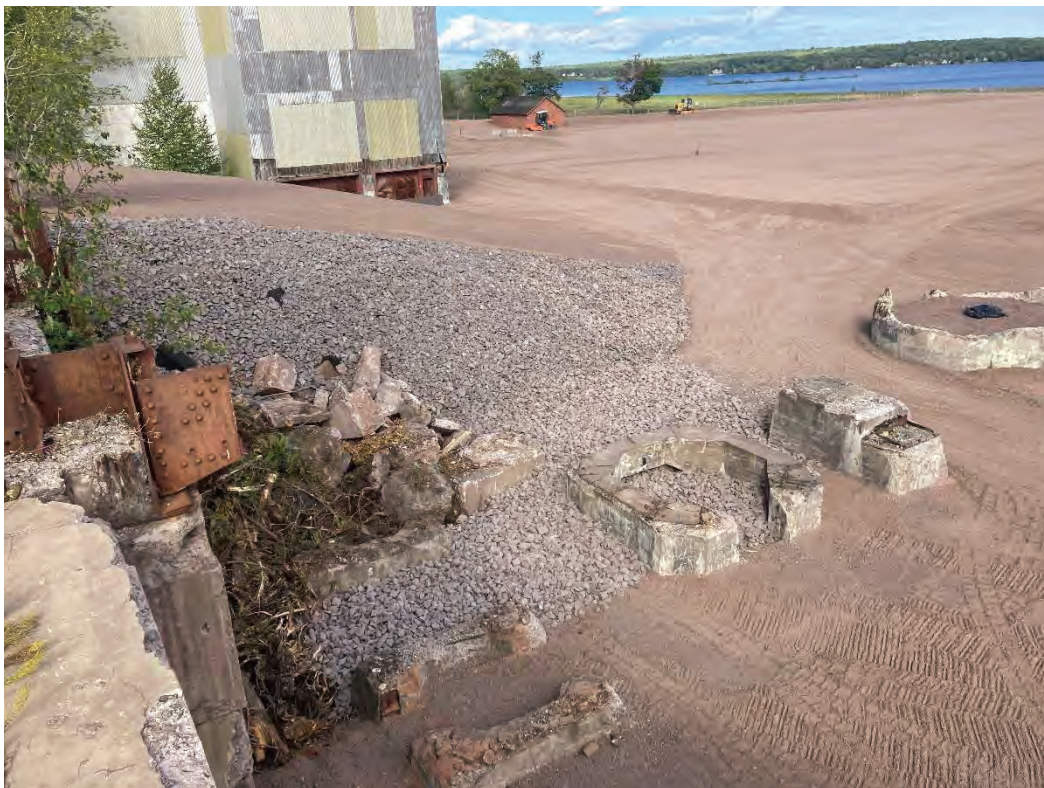
Base of the consolidation pile with final riprap (facing east) 2020
