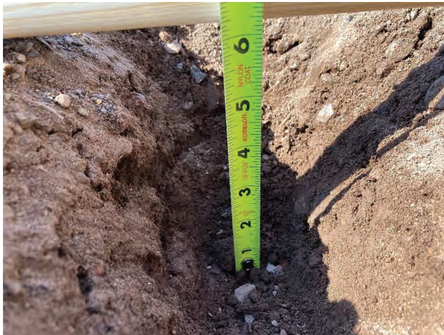
Completing 22A thickness quality control checks (facing south) 2020
