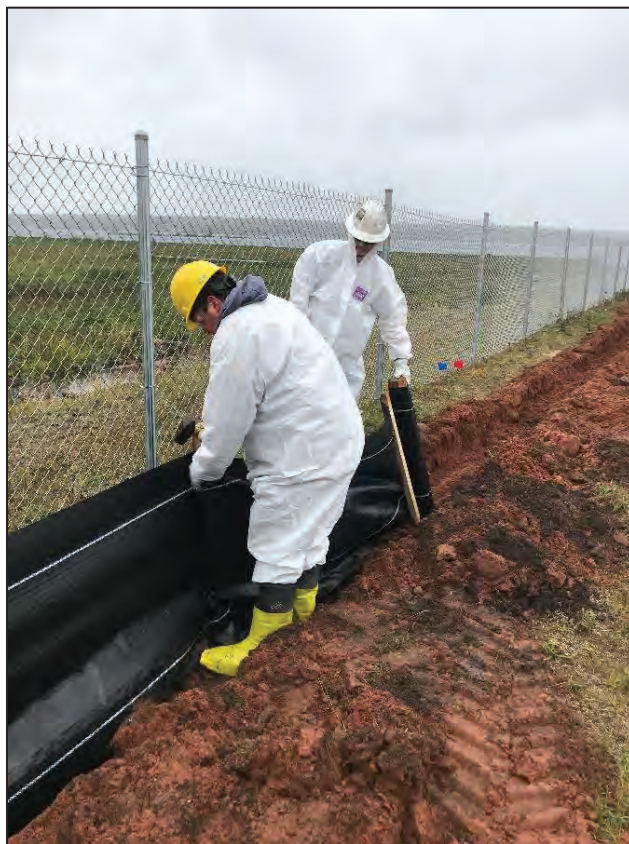
Soil Erosion and Sediment Control (SESC) Plan Implementation: Silt Fence installment in lead contaminated area (facing Southwest) 2019
