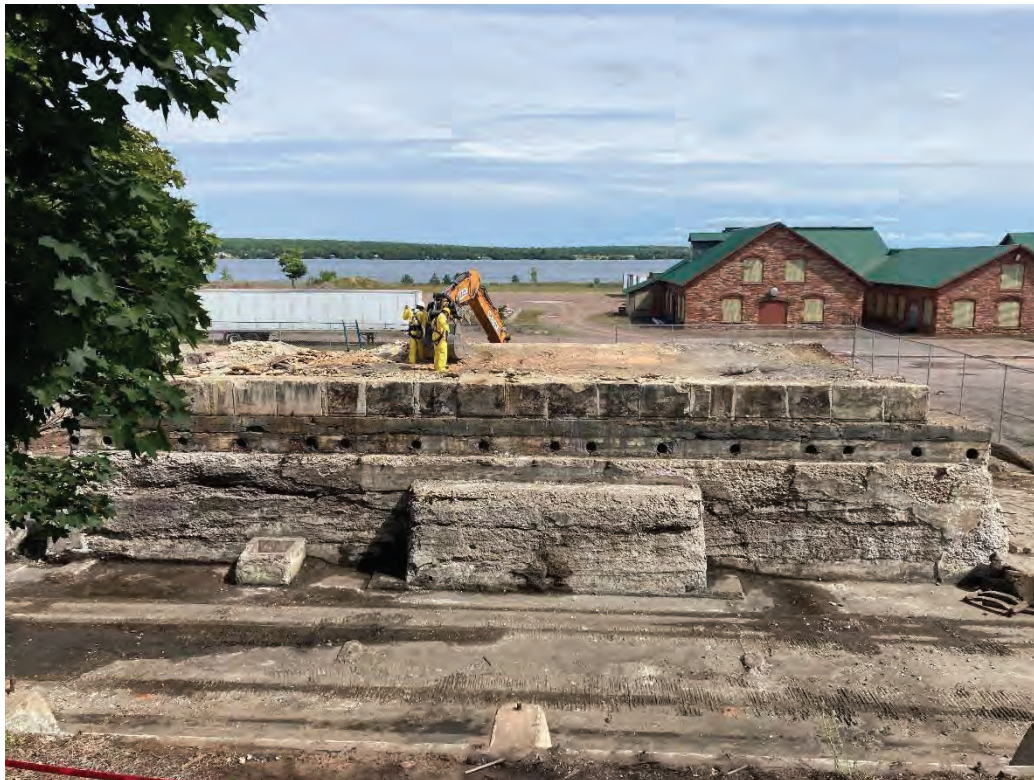
Cleaning elevated foundation using the “dead stick” excavator as a tie off (facing southeast) 2020
