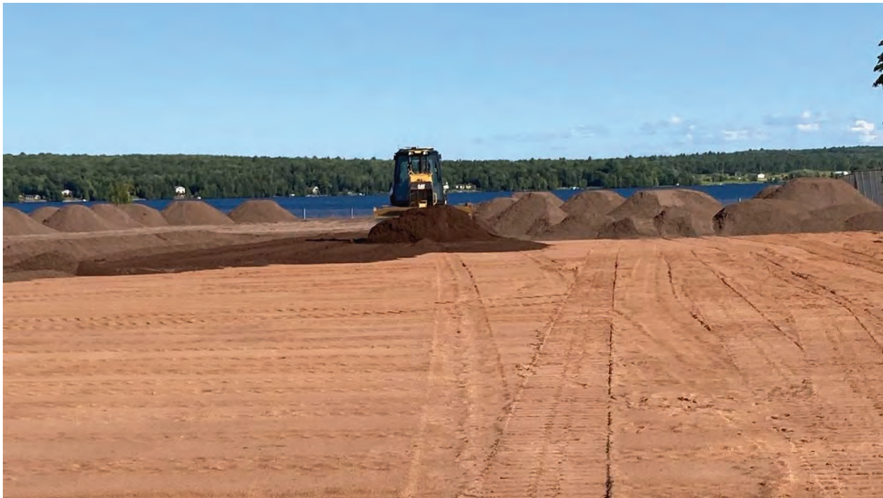
Pushing out delivered 22A gravel over the compacted sand (facing east)
