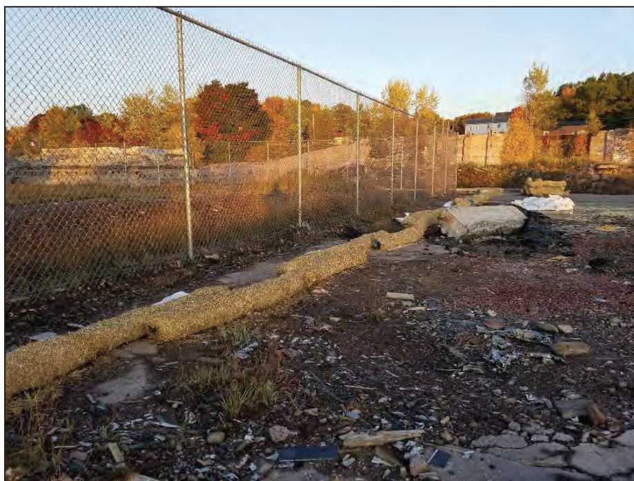
SESC Straw waddle placement along the fenced perimeter (facing northwest) 2019
