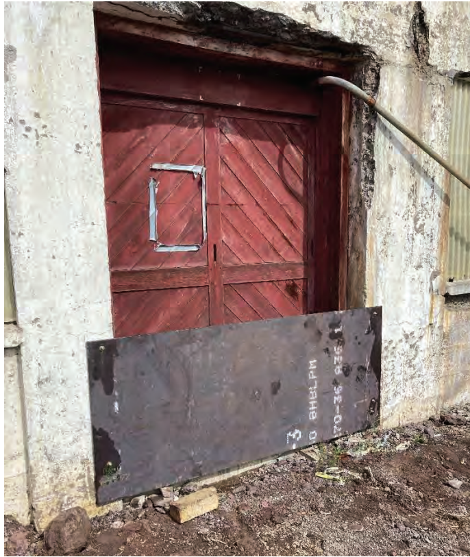
Steel secured at Mineral Building doorways to hold fill out of the building (facing north) 2020
