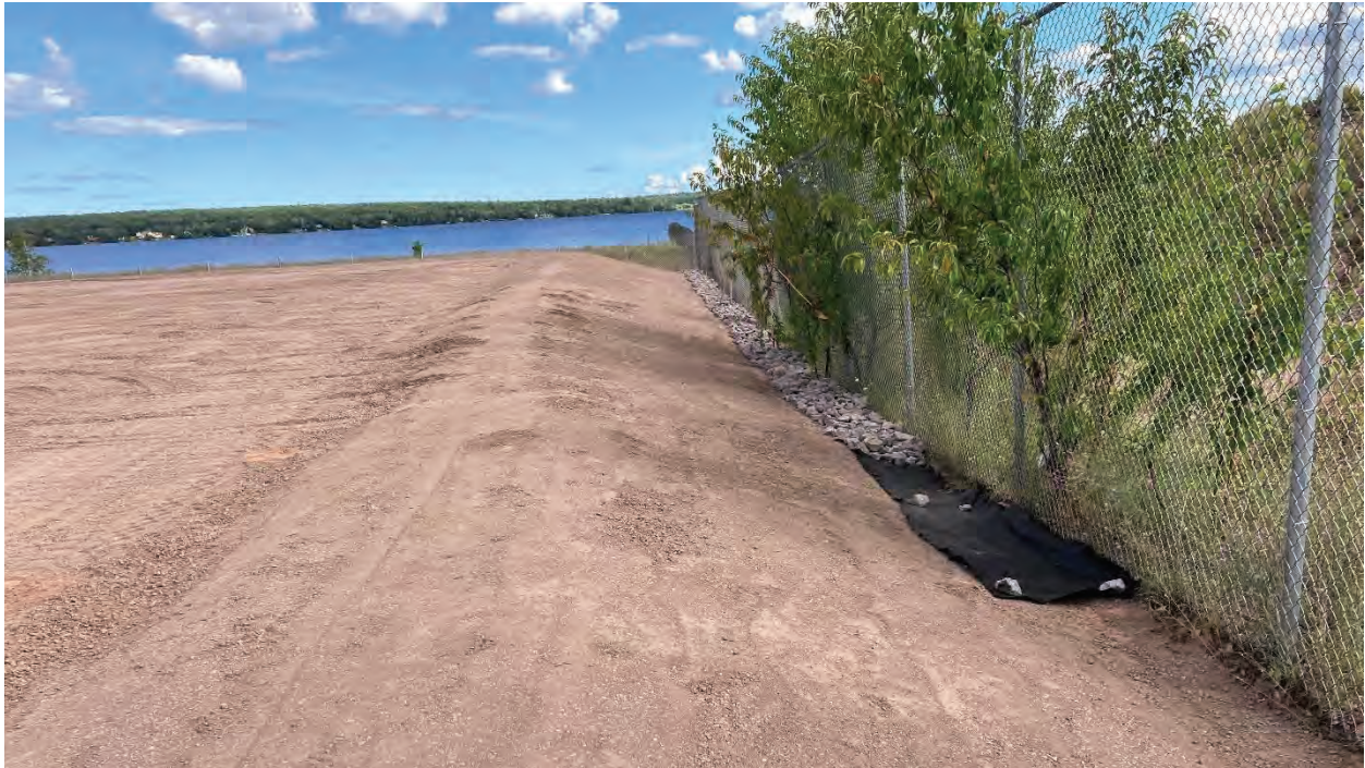
Placing riprap along the south fence line near the southeast corner of the site (facing southeast) 2020
