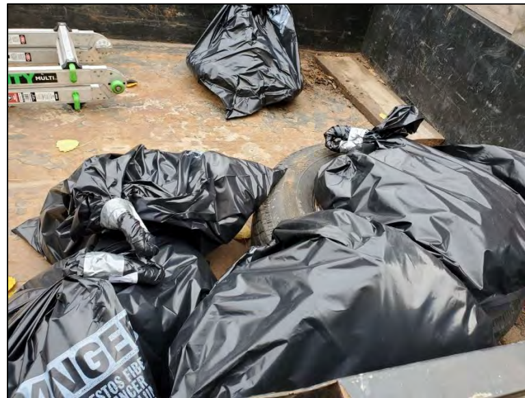
Photo 6: View of the five bags of ACBM roofing and SACM tar with fibers removed from the Coal Dock Burn Area.
