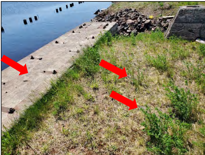
Photo 3: View of suspect ACBM tar with fibers (red arrows), which is flaking off the concrete bulkhead onto the capped area of the Coal Dock Burn Area.
