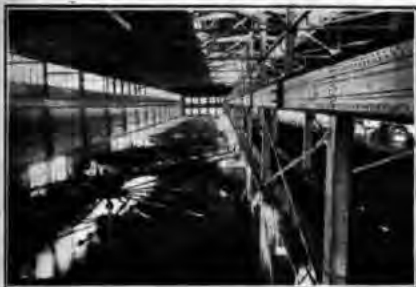
Row of tanks in leaching plant. First tank has launder and distributor in place. Second tank is uncovered. Others have covers in place.
