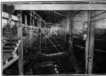
Leaching plant, showing "V" settling tanks, Dorr quadruplex classifier, and leaching tanks with covers in place. Colored lights against column in foreground are signals flashed from plant to plant to show load conditions.
