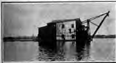
Dredge and portion of pontoon line
