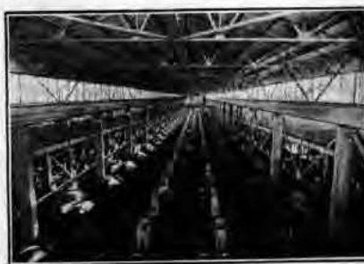
Regrinding plant, showing 64 8-ft. x 18-in. Hardinge mills
