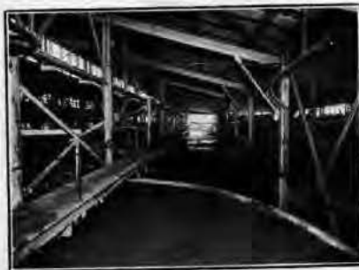
Flotation plant, showing row of Dorr thickeners. At the right are the backs of the flotation machines.
