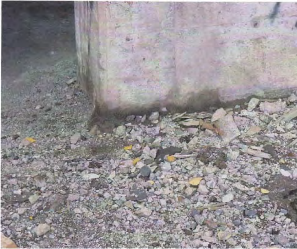
11. Photo shows door jam sample location (looking west)
