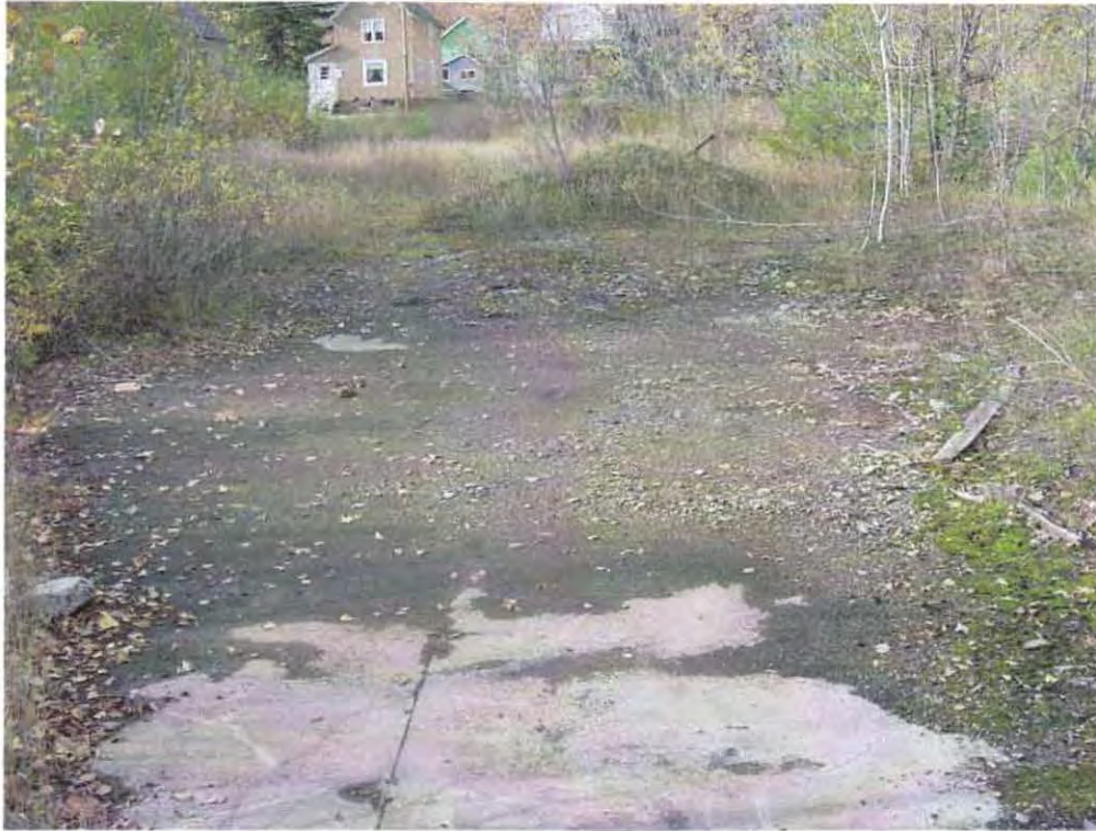
5. Photo shows concrete floor location (looking northwest).
