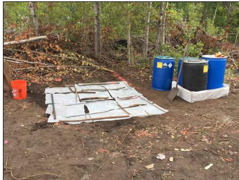
Photo 6: View looking north at a grid of plastic sheeting set up to screen soil for the presence of mercury during excavation.
