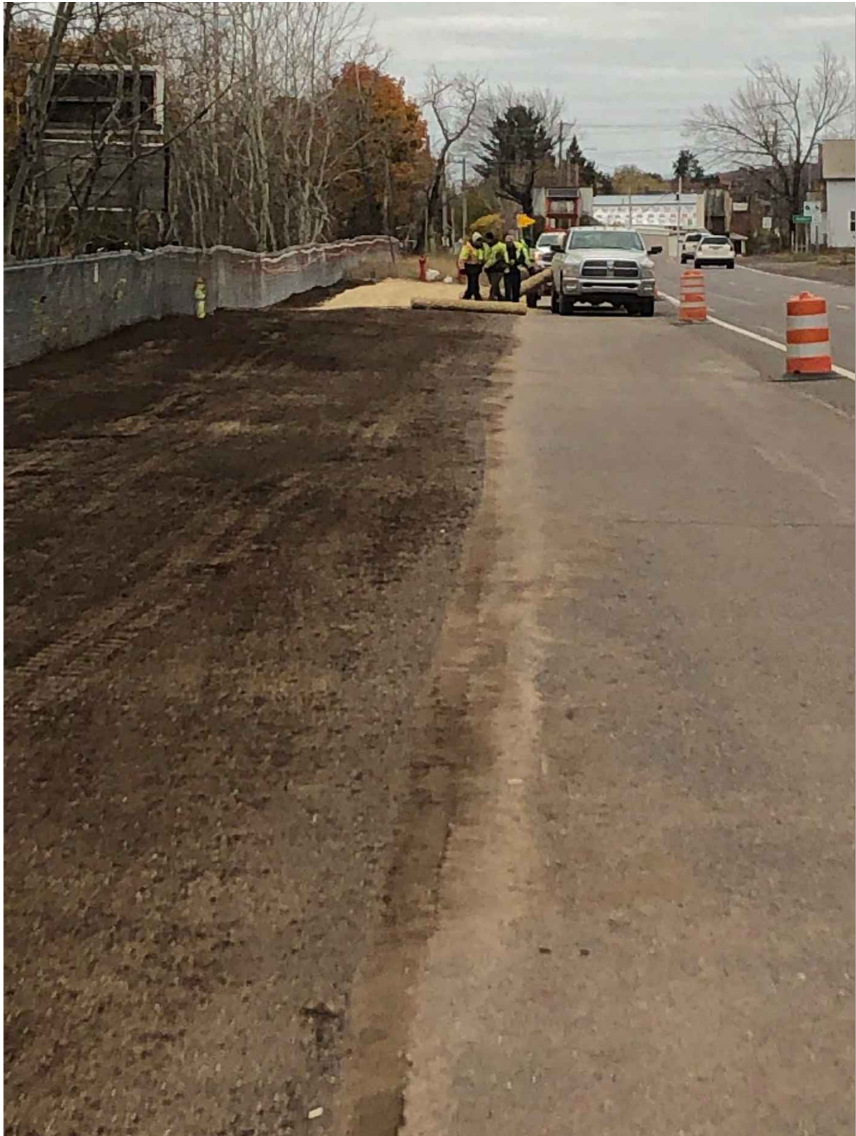
Photo 5: Installation of Mulch Blankets
