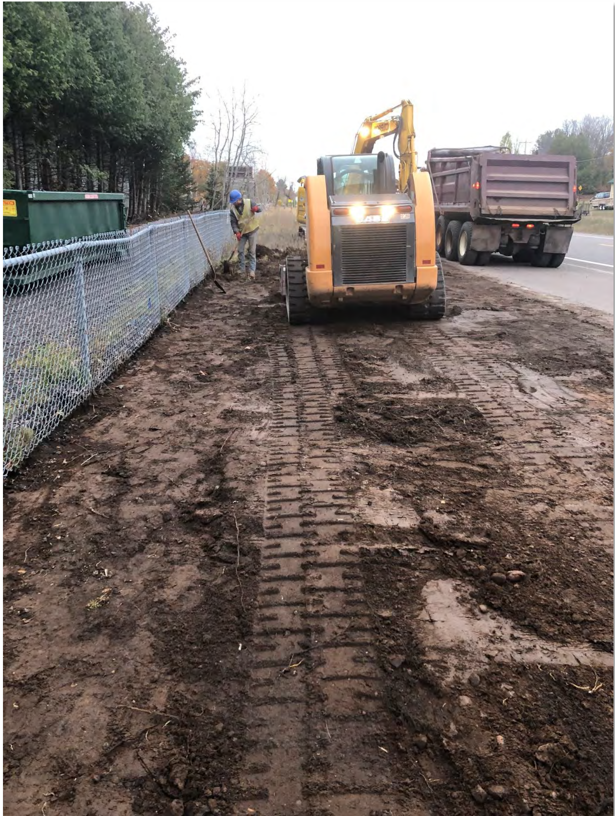
Photo 2: ROW Soil Excavation and Soil Removal Along Fence line
