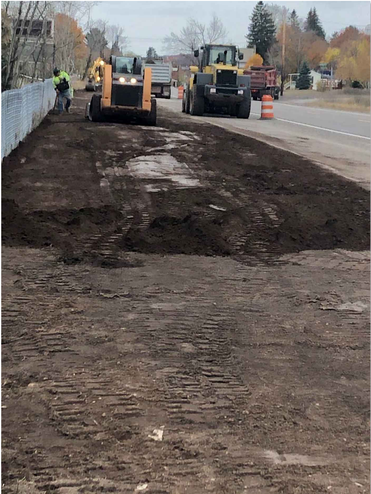
Photo 3: Placement of Topsoil
