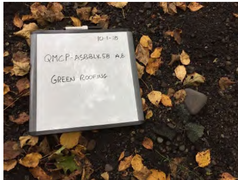
Photo 2: View of green roofing material, sampled as QMCP-ASBBLK58. Photo taken 10/1/2018.
