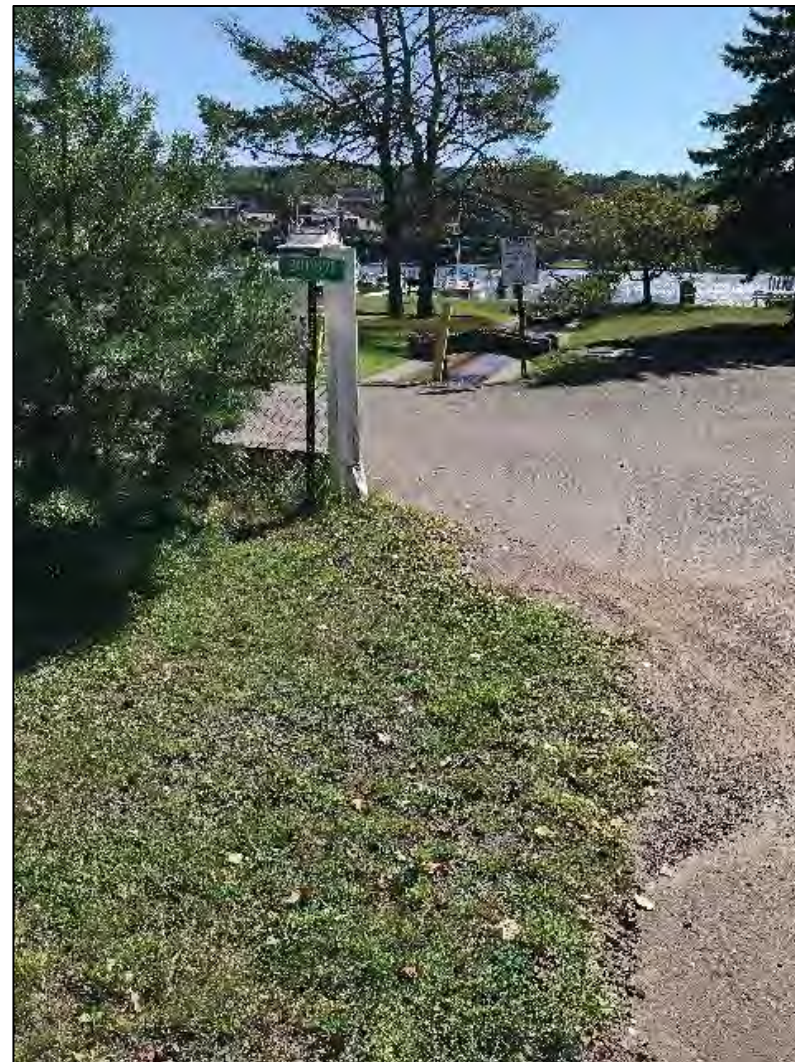
Photo 2: View looking south of the open channel discharge to the Portage Canal identified as Observation Number Outfall001. Photo taken 9/13/2018.
