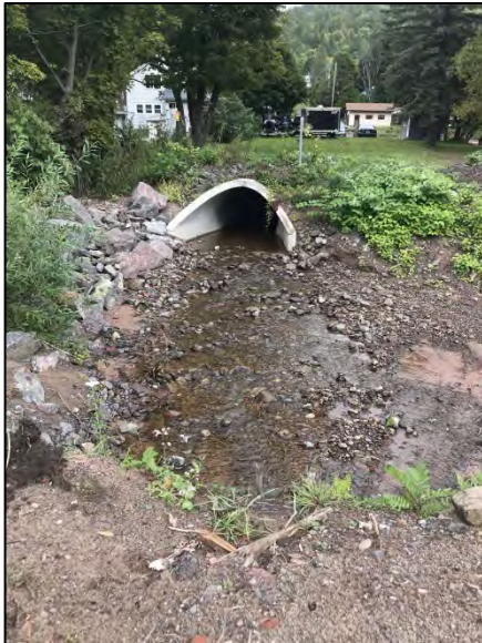
Photo 3: View of a culvert outlet north of the Trail ROW in Area E. Photo taken 9/25/2018.
