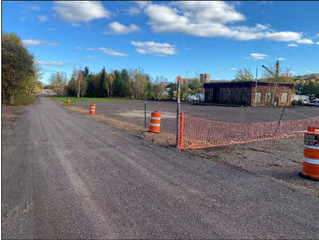
Photo 1: View looking southeast of the designated trail through the Julio Salvage Parcel following MDNR's grading and graveling, and Priority Area 1 following EPA's removal and placement of gravel cover including a vegetated buffer adjacent to the south side of the designated trail.
