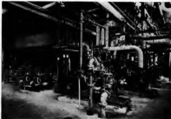
Figure 6. Ahmeek Mill Boiler House. Control compressors, ash pump and boiler feed pump.
