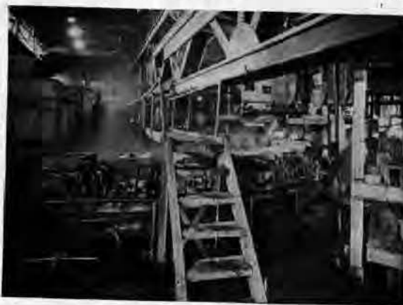
Figure 9. Clark casting wheel
