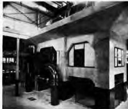
Figure 9. Ahmeek Mill Power House, No. 8 turbine room, showing reinforced concrete turbine foundation and condenser.
