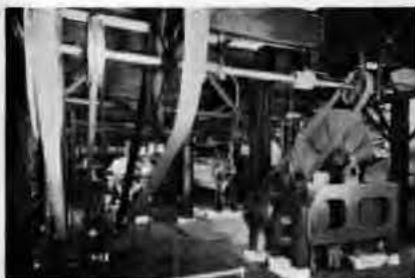
Figure 10. Vacuum and pressure filters in still house, Lake Linden
