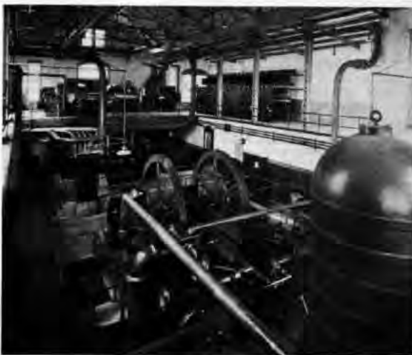
Figure 11. Ahmeek Mill Pump and Turbine Room. In the foreground is the 28,000-g. p. m. triple expansion reciprocating pump. On the same floor is the No. 7, 1,250-kw. reducing turbine unit and the by-pass reducing valves. In the rear is the No. 6 2,000-kw. exhaust steam turbine unit and the 2,300-volt switchboard.
