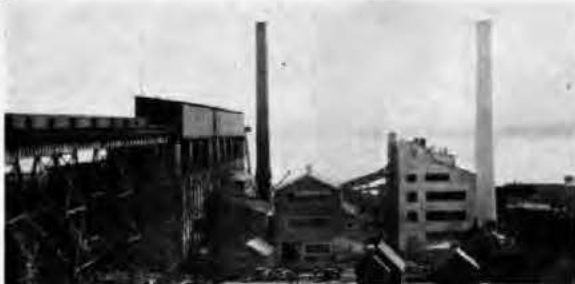
Figure 3. Ahmeek Mill and Power Plant, looking east. Above the concrete are the steel ore bins served by a double track. Coal chutes under the rear track lead to coal bins built into the concrete supporting structure.
