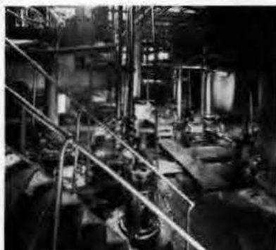
Figure 7. Ammonia solution pumps in leaching plant, Lake Linden
