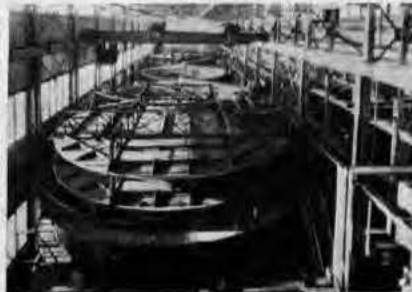
Figure 16. Ammonia leaching tanks, Tamarack reclamation plant.
