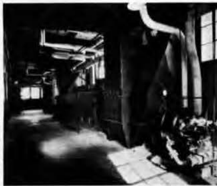
Figure 5. Ahmeek Mill Boiler House. Forced draft fans with steam turbine drives.
