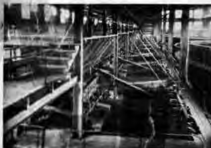
Figure 5. Leaching plant classifying system, Lake Linden
