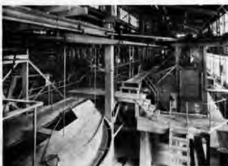
Figure 2. Standard minerals separation flotation machines, north flotation plant, Lake Linden.
