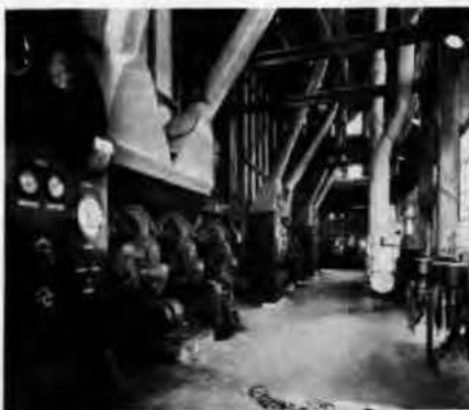
Figure 4. Ahmeek Mill Boiler House. Operating floor showing stokers, main steam piping and control panels.
