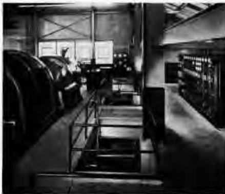
Figure 8. Ahmeek Mill Power House, No. 8 steam turbine generator unit with its 13,600-volt switchboard.
