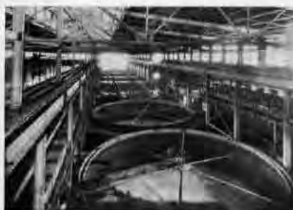
Figure 6. Sand leaching tanks in leaching plant, Lake Linden
