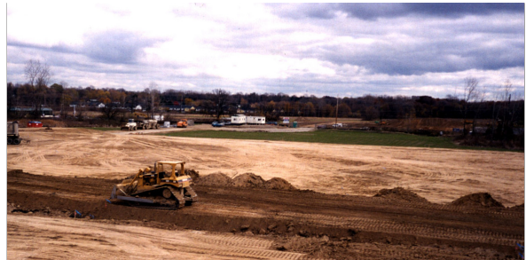
Construction of a soil cover (exposure barrier) over the former Linden Road Landfill in Flint Charter Township (Genesee Co.).
