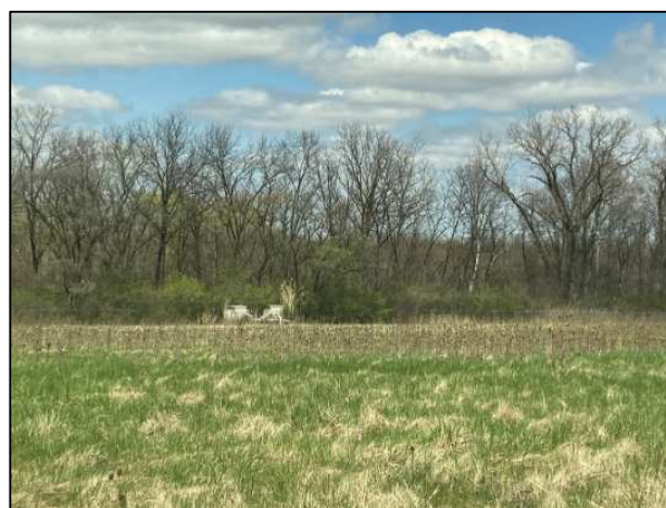
Grass cover and leachate collection “wet well” on the north side of the Old Wayne Landfill, facing north.
