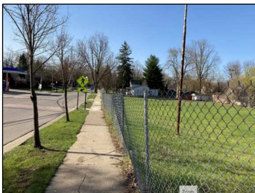
Federal Screw Works - View of fence running along eastern edge of the property showing the fence in poor condition – leaning, separated from supports. Photo taken looking south.
