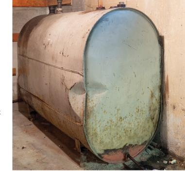
**Closing a Tank:** In the event your heating oil tank is no longer used, the tank must be taken out of service and properly closed. Proper closure for both an AST and UST is defined as emptying the tank and related piping of heating oil. After the oil is drained, the tank must be properly cleaned to remove all vapors and residual oil. Once the AST has been emptied and cleaned and there is no evidence that the tank leaked, the tank is considered closed and can be removed.
