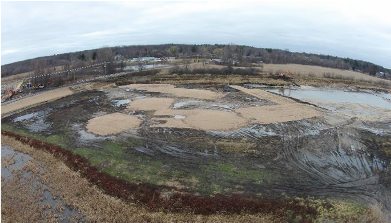
Figure 3. Final grade and habitat islands in the East Pond, looking northeast.
