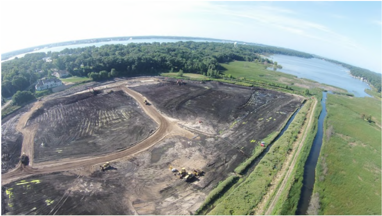
Figure 2. Site construction in the West Pond, looking south at Bear Lake.
