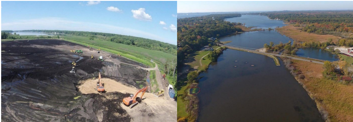
Figure 4. Bear Creek restoration removal of sediments (left) and post-restoration after berm removal (right).
