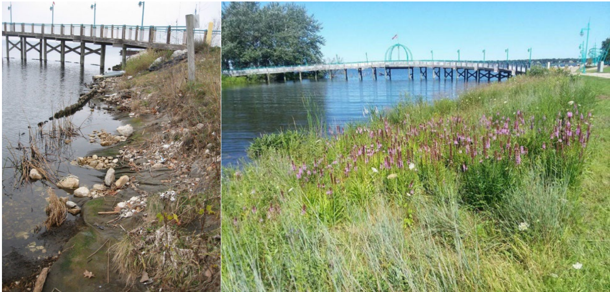
Figure 10. Heritage Bay before restoration facing north toward Muskegon Lake (left) and after restoration facing south into the inlet (right).
