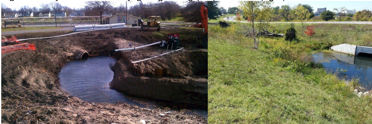
Figure 18. Ryerson Creek daylighting during (left) and after (right).
