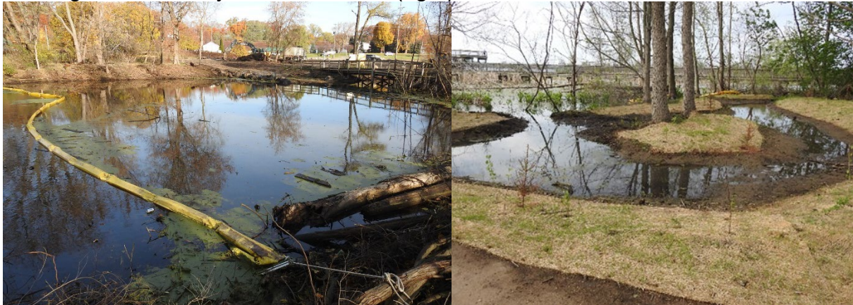
Figure 14. Nature preserve during wetland drawdown (left) and after drawdown. Muskegon Lake is beyond the tree line (right).
