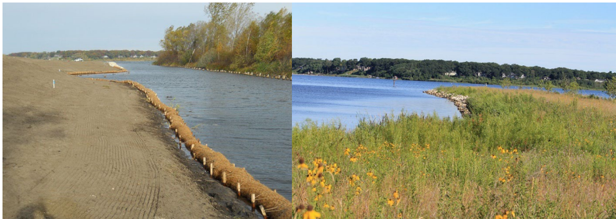
Figure 7. Foundry Park during restoration after fill removal and before planting (left) and after restoration (right).
