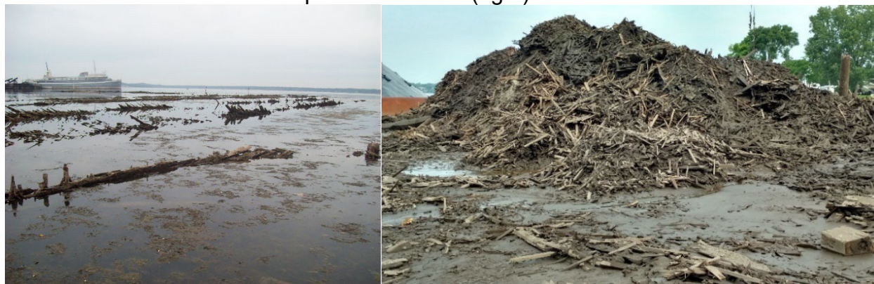
Figure 13. Mill debris before removal facing west in Muskegon Lake (left) and after removal when mill debris was placed on shore (right).
