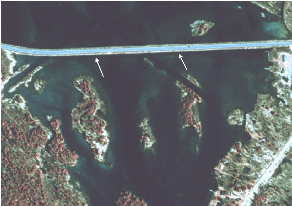
Figure 2. Closeup of the causeway. Presently, two, six-foot culverts, indicated by the arrows, are the only flow remaining.
