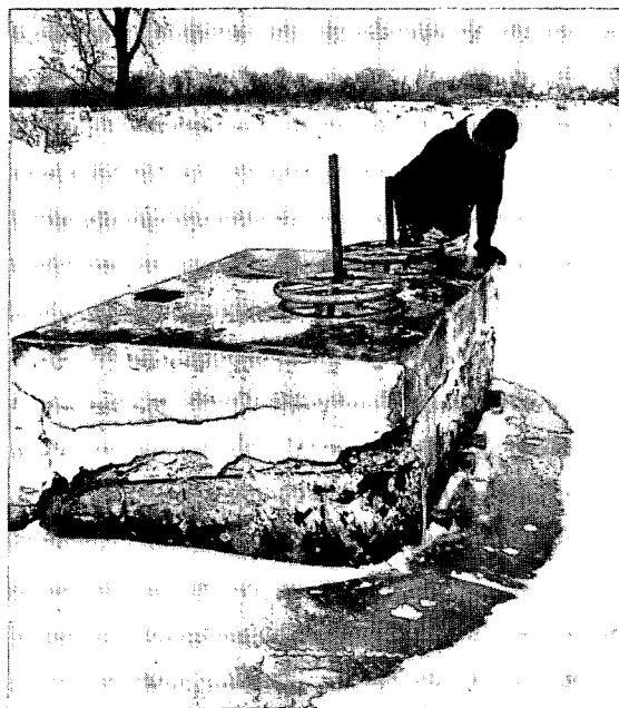
Left: Concrete deterioration caused by weathering.
