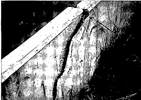
Right: Structural crack caused by wall movement.
