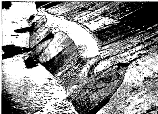
"Piping" in progress. Note bales of straw for plugging "pipe."
