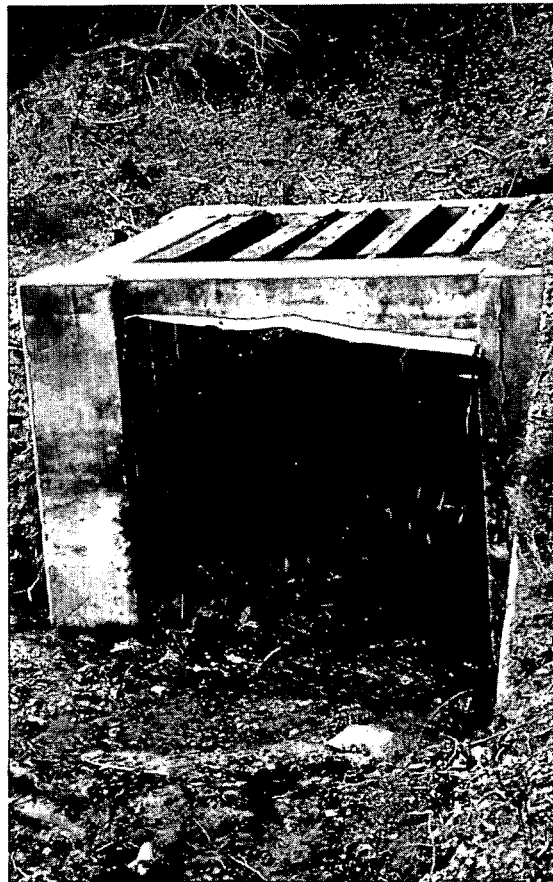
TRASHRACKS ON PIPE SPILLWAYS
