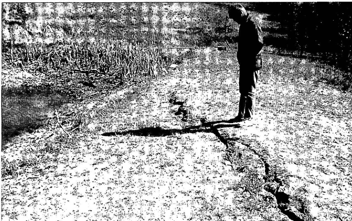
Longitudinal crack.
