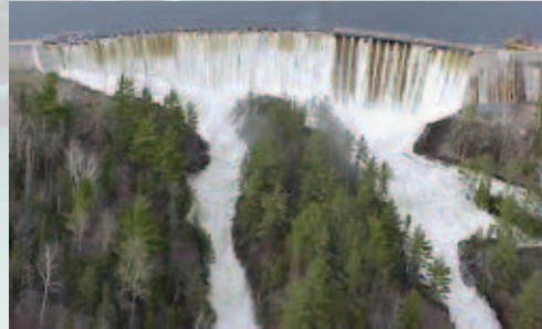
FIGURE 3: When the fuse plug in Silver Lake Dam failed, more than nine billion gallons of water unexpectedly rushed out of the reservoir and over Hoist Dam. No lives were lost and no major injuries occurred – thanks to an updated emergency action plan and a coordinated response of the part of all involved.
