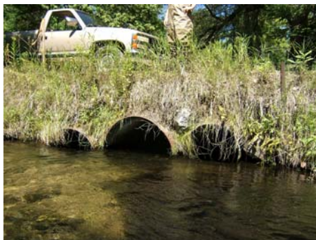
Figure 4. Green River at Green River Road looking downstream at the road.
