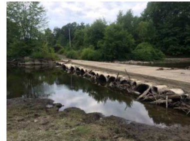
Brick Plant Bridge, August 2015
