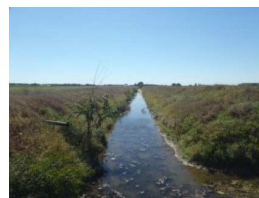
Carson Drain (Ryan Road) 2015
