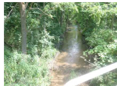
Pratt Drain (Geek Road) 2015
