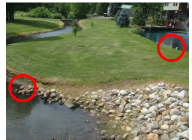
Marion Genoa Drain looking at downstream location of pipe
