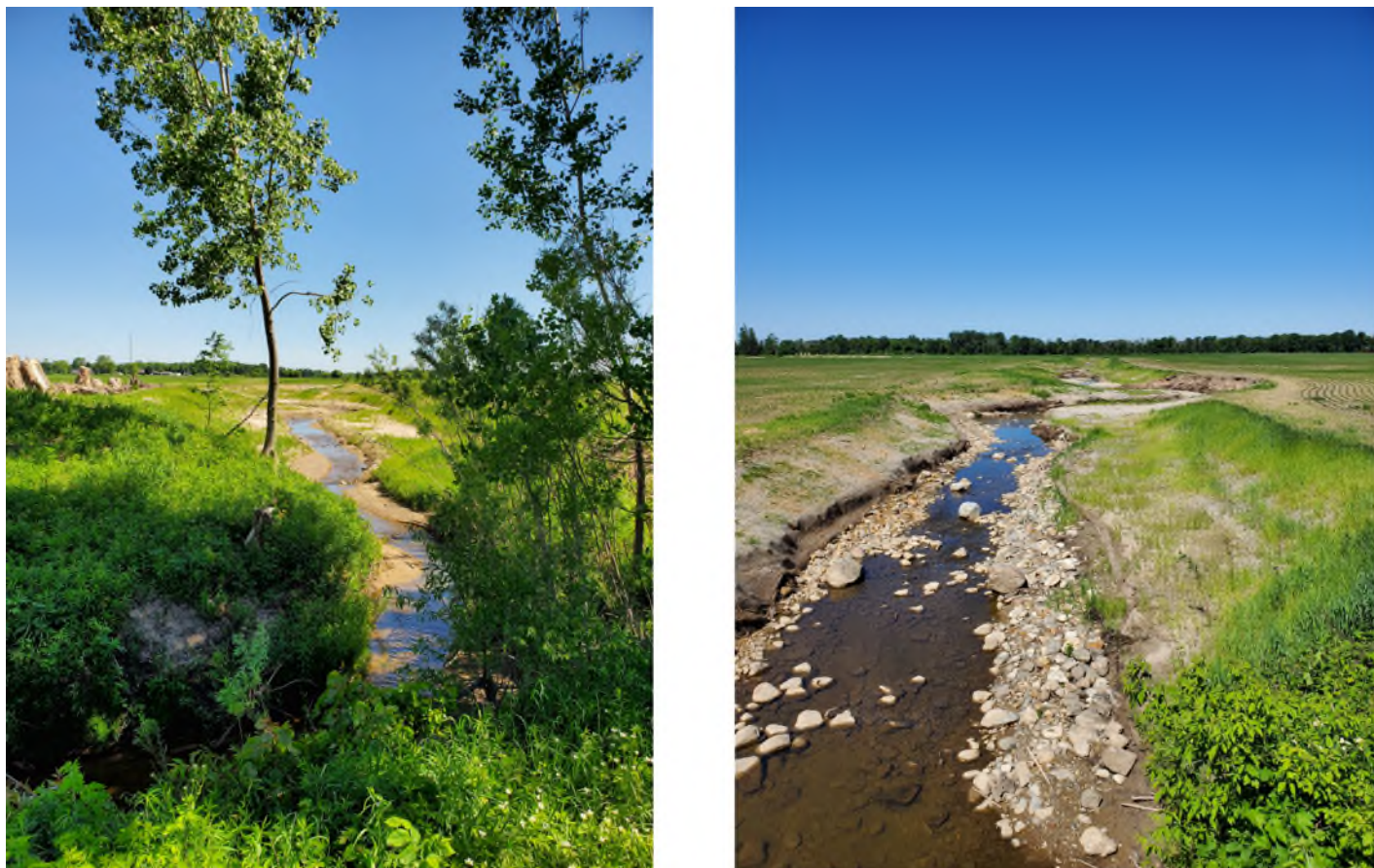
Figure 10. Two-stage ditch banks at Wilson Street site (left photo) and slightly upstream (right photo) in June 2020.
