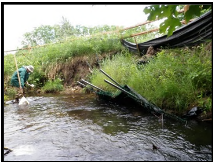
Photo 22. 2019 view from stream. Berm/stream bank is failing.
