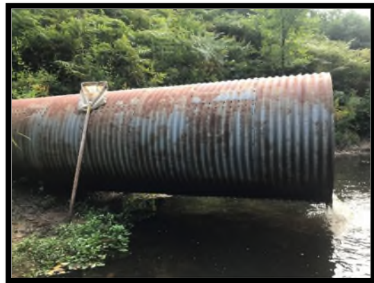
Photo 27. Claybanks Creek downstream of Pine Creek Road, August 2019. Image is a perched culvert.
