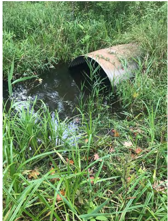
Photo 7. Peterson Creek at S7 Road, note undersized culvert in relation to stream size.
