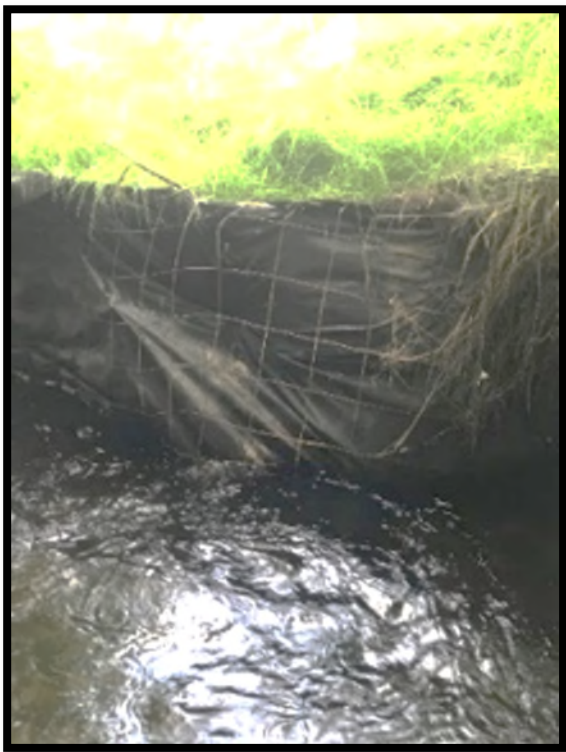
Photo 20. 2014 view from stream. Berm/streambank failing.
