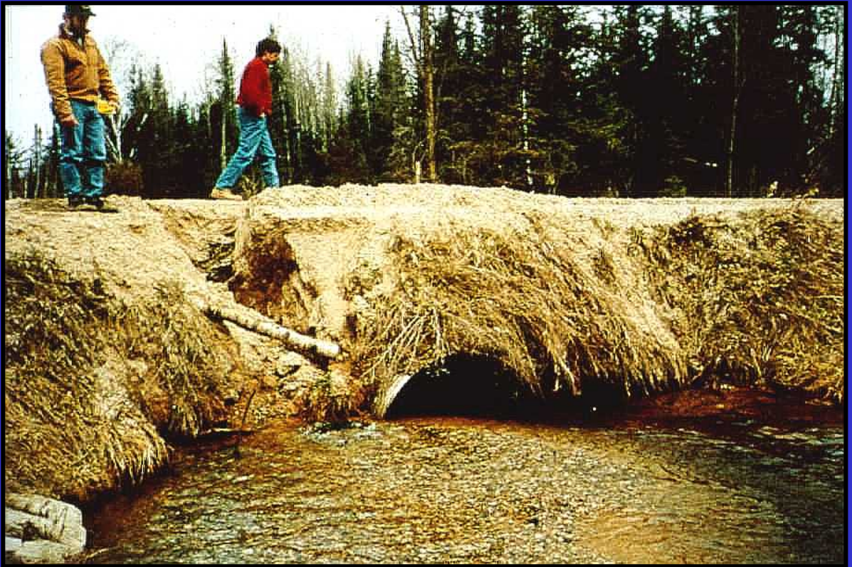
Figure 1. Kulka Creek crossing near Grayling, Michigan. (Before)
