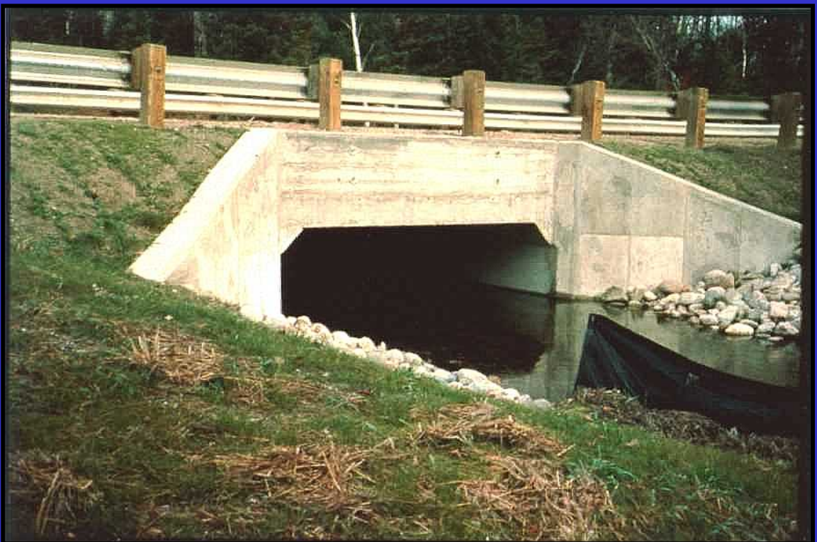
Figure 2. Kulka Creek Box Culvert Replacement (After)
