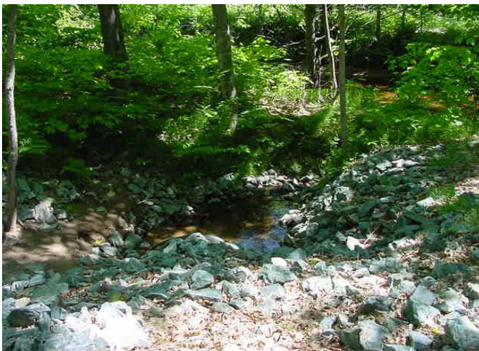
Yellow Dog at Bear Lake Site After: Yellow Dog site with water diversion practice implemented.
