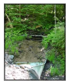
A new, extended culvert (viewed from the top) allows water to flow more freely under CO Rd 510. This site features a pan to direct water out of the culvert toward the stream bed.
