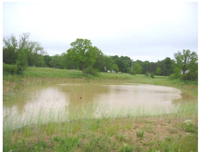
Description: Infiltration Basin immediately after a rain event, which receives water from the diversion structure at a rate of 30 cubic feet per second.
