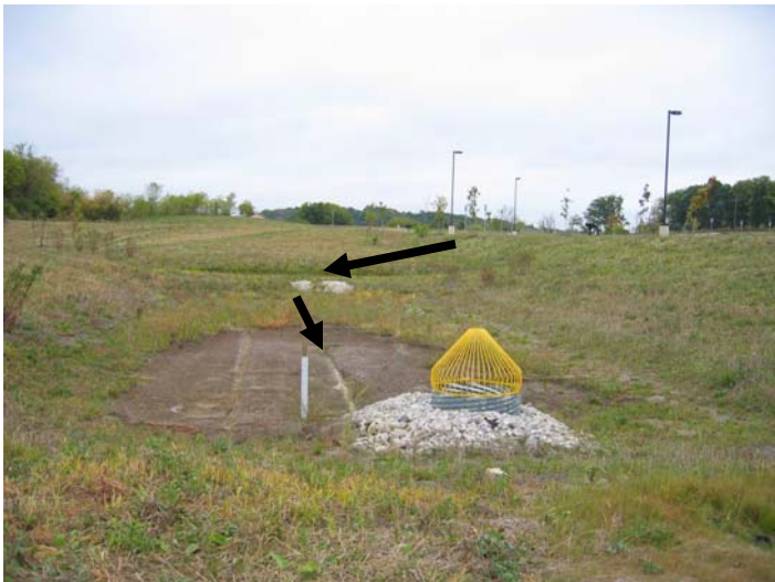
Above: The entrance to the Storm water Demonstration Park. Water flows to modular pavement, which promotes infiltration. Top Right: Traditional pavement on right draining into an infiltration area. Lower Right: Native vegetation used throughout the park to soak up storm water.
