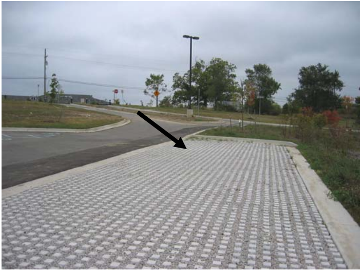
Above: The entrance to the Storm water Demonstration Park. Water flows to modular pavement, which promotes infiltration. Top Right: Traditional pavement on right draining into an infiltration area. Lower Right: Native vegetation used throughout the park to soak up storm water.
