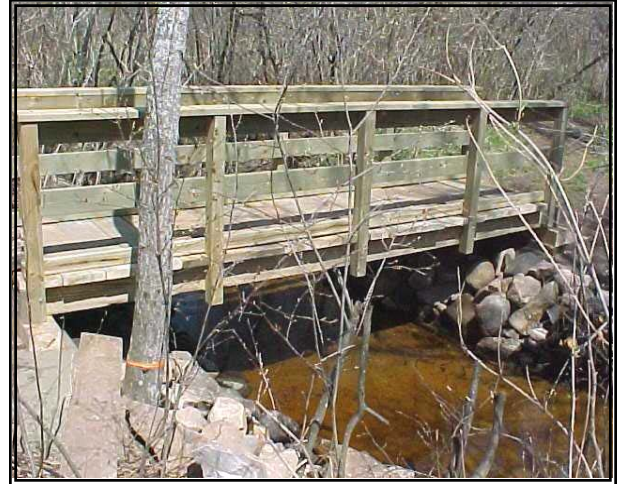
Hosking Creek Bridge After:
