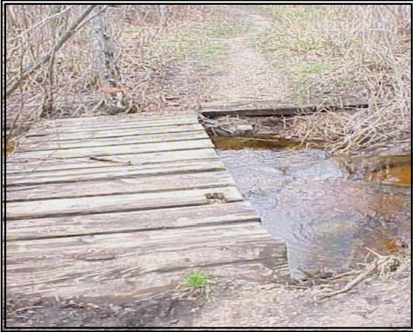
Hosking Creek Bridge Before:
