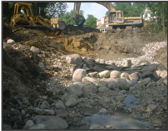
Summer 2002: Step Pools during Construction
