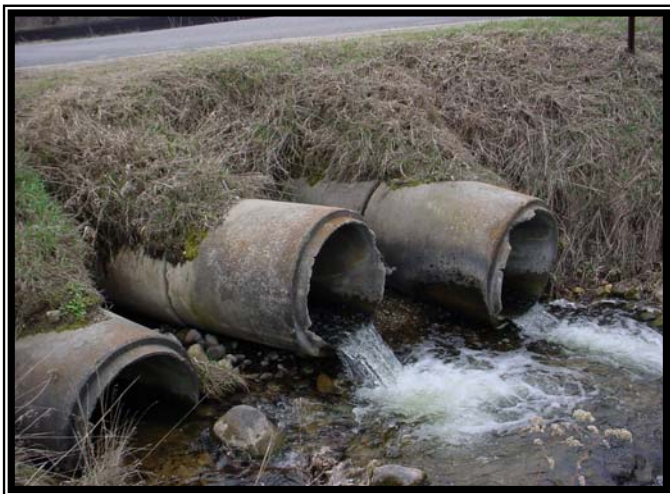
Road Stream Crossing Before
