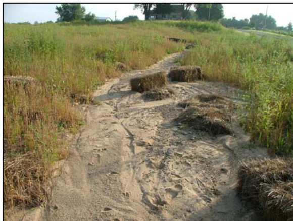
Devenney Farm - before construction, of grassed waterway. Active erosion occurring.
