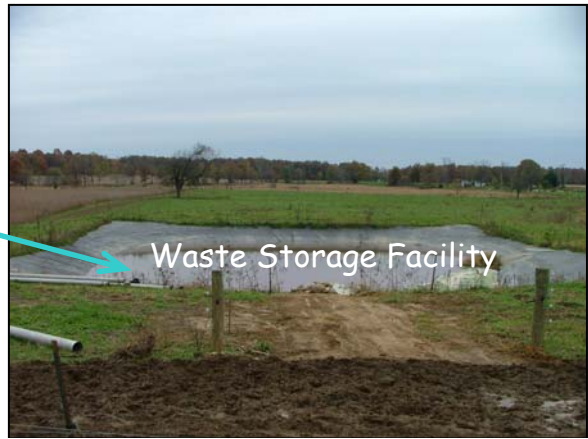
MarGro Farm - after construction, existing waste storage facility was connected to silage runoff collection basin.
