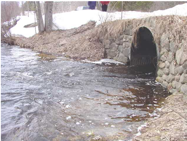
Site #B-18 Before: Both road crossing sites, #B-18 and #B-17, had 5' diameter culverts on a 20' wide stream, the Little Betsie. The sites were even on the same road. Pool formation, scouring and embankment erosion were major problems.
