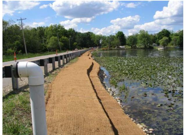
**Beadle Lake Shoreline After Construction of BMPs:** BMPs included construction of a glacial stone toe along the entire 520 feet of road frontage. On top of the stone toe, soil was backfilled into a wrap of bioengineered materials to create two successions of shoreline. The fill material was densely seeded with a native wildflower mix.
