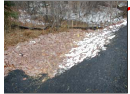
Site #8 - CR 510, Midway Creek (after). Elimination of sand berm. Road was paved and storm water rerouted into the re-sloped ditch with a water diversion at the end to dissipate the flow of runoff.
