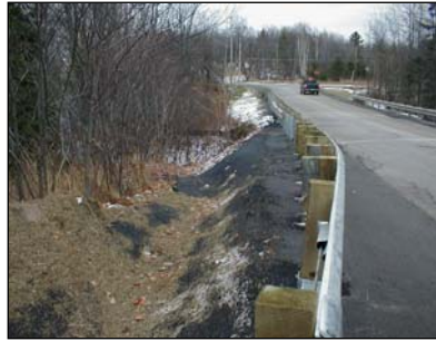
Site #8 - CR 510, Midway Creek (before). Sand from roadway was bermed up along railing support. Sediment was being directly deposited into the stream.
