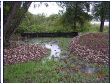
Filtering water from storm event
