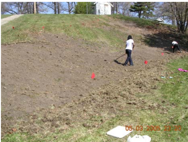
Hillside erosion on west side of creek
