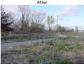
Roadway removed and replaced with 6' wide gravel walking path and disturbed areas replanted with native perrenials.
