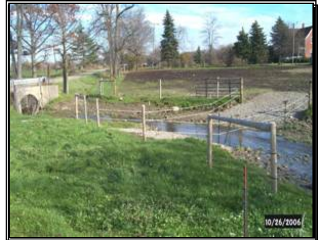
The same site on the O'Loughlin Drain shortly after the livestock crossings and fence was installed. The banks were still not vegetated at this time.
