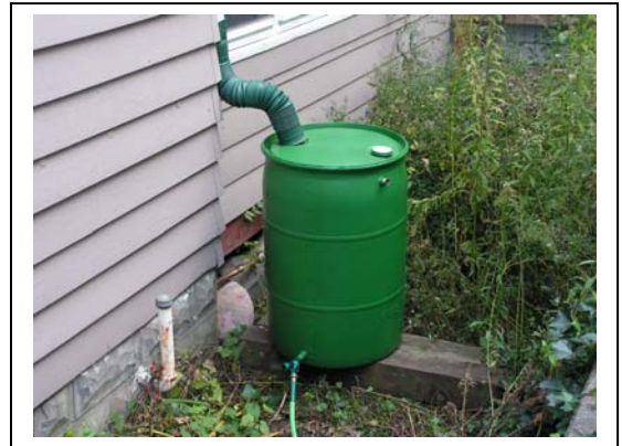
Hillcrest Neighborhood After: Completed, installed rain barrel.
