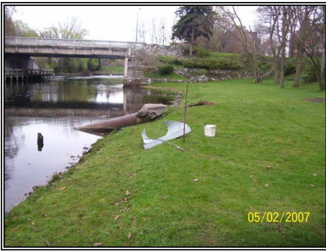
Hannah Park Restoration Project - Boardman River: Top left - before picture showing lack of riparian buffer, eroding banks, and failing stormwater outlets. Right (clockwise from top-left) - Riparian buffer, fishing platform (quarried rock), bank stabilization; stormwater outfall; Oil/Grit Separator at west end of park (Aquaswirl Unit); Wooden fishing platform and stormwater outfall.
