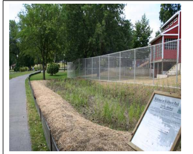
Bioswale – after planting. Showing new fencing that keeps animals out of area that directly drains to the Rocky.
