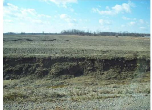
Erosion and sedimentation is very common to the watershed due to the lack of environmental stewardship. This picture shows how a ditch was improperly dug out and not stabilized (reseeded), causing the banks to slump and erode away. Also, you will notice this field is worked up to the edge of this ditch, with no buffer protect it.
